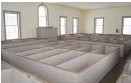
Having served a number of different denominations over the years, the Free Meeting House in Moncton was restored to its earliest, 1821 interior configuration by following floor marks and other physical and documented evidence. Missing features from the selected restoration period were replaced.
