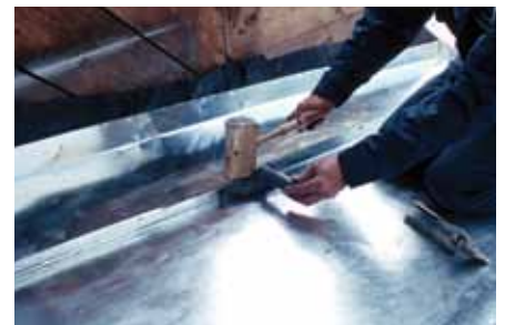
When restoring the former post office in Dawson, YK, the metal roofing surface, which was too deteriorated to repair, was replaced in kind. Physical evidence from the restoration period was used as a model to reproduce the characteristic standing seam detail.
