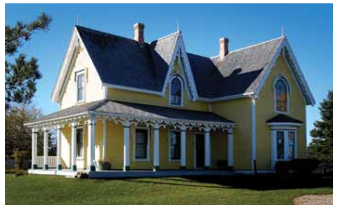
Based on documentary evidence, including an 1880 engraving, the original fenestration of the Biddeford Parsonage Museum in P.E.I. was restored and roof finials replaced.
