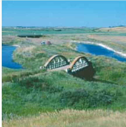
The Eagle Creek Cement Bridge in Saskatchewan is a good example of the nearly 90 reinforced concrete bowstring bridges that were constructed during the 1920s and 1930s as part of a comprehensive road building program in southern Saskatchewan. The graceful bowstring arches of these bridges, which blended functional engineering technology with aesthetically pleasing design, are character-defining elements. Repair or replacement of any parts of the bowstring arches should carefully designed for compatibility, matching the original form, materials and detailing of the arches.
