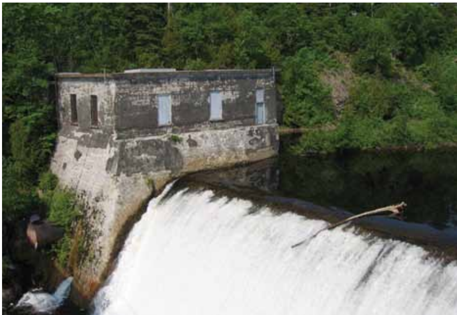
Remains of hydroelectric installations.
