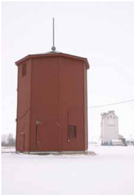
Completed in 1904, the tall wood frame Clearwater Canadian Pacific Railway Water Tower in Manitoba is an excellent example of an intact railway water tower. Twelve thick timbers are set on concrete bases and are strengthened with cross-braces that support the cedar-lined water tank, which occupies the top half of the structure. The water tower retains many of the original pipes, valves and controls used in filling and using the tank. When ceasing operation at a work such as this, the character defining pipes, valves and controls should continue to be subjected to regular maintenance to prevent their deterioration.
