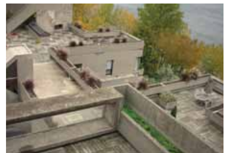
The character-defining elements of Habitat 67 in Montreal include modern urban concrete furniture. These built features of the landscape complement and reinforce the building's forms, materials and colour.
