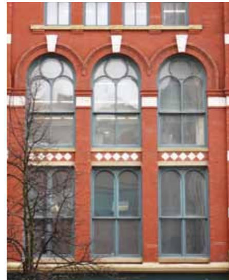
These large windows on King Street in St. John were originally slated for removal and replacement as part of the CentreBeam Place rehabilitation project. Instead, a condition revealed that the original windows could be retained and repaired, with the addition of interior storm to meet energy efficiency requirements.
