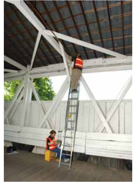
Before beginning project work, the form, materials and condition of engineering works should be documented. Heritage recording of the Powerscourt Covered Bridge, National Historic Site of Canada in Powerscourt, QC, the only surviving bridge that uses the McCallum inflexible arch construction, included detailed measurements and a photographic record.
