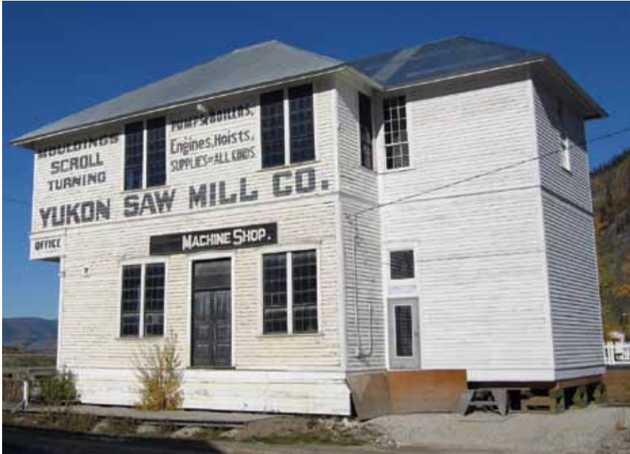
A compatible addition to the rear of the Yukon Sawmill Co. Office provides space for services. If necessary, it could be removed without affecting the building's historic fabric. One window opening and the surrounding wall framing were altered to provide space for a connecting door.
