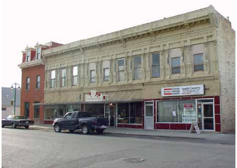
Before rehabilitation: east façade, looking southwest.
