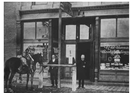
Circa 1910 photograph of Grier Block storefront, south bay. Photographs like this were an indispensable resource in developing the storefront restoration plans.
