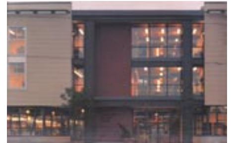
A study of the area's historic warehouses will lead to suitable contemporary interpretations of this common building type.
