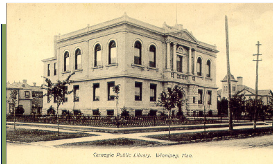
Carnegie Library, home of the Archives and Records Control Branch, 380 William, circa 1908.
