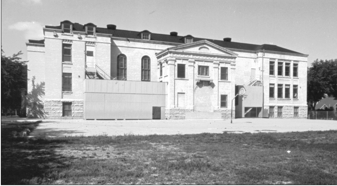
Plate 4 – Laura Secord School, rear façade, 1970. (Courtesy of the Provincial Archives of Manitoba, Architectural Survey. )
