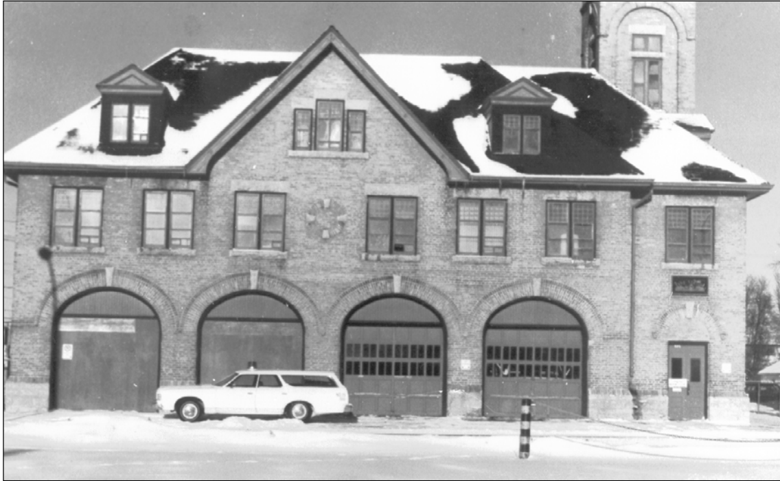
Plate 1 – Former Fire Hall No. 8, 325 Talbot Avenue, as an ambulance depot, 1981. (Courtesy of the Western Canada Pictorial Index, A538-17140. )
