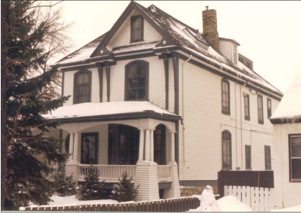
Plate 1 – John C. Graham House, 137 Scott Street, front (east) and side (north) façades, 1988. (M. Peterson, 1988.)
