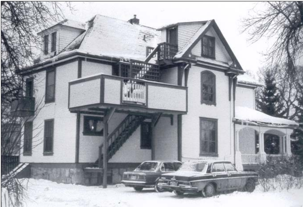
Plate 2 – J.C. Graham House, side (south) and rear (west) façades, 1988. (M. Peterson, 1988.)
