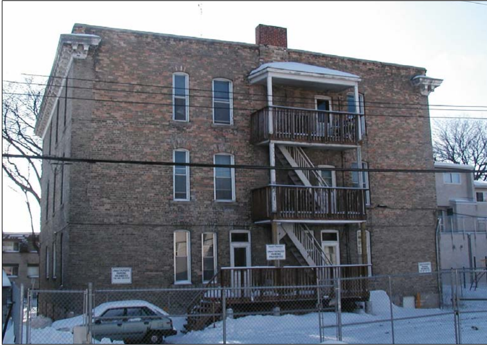
Plate 5 – Rear (north) façade, 2005. ( M. Peterson, 2005. )
