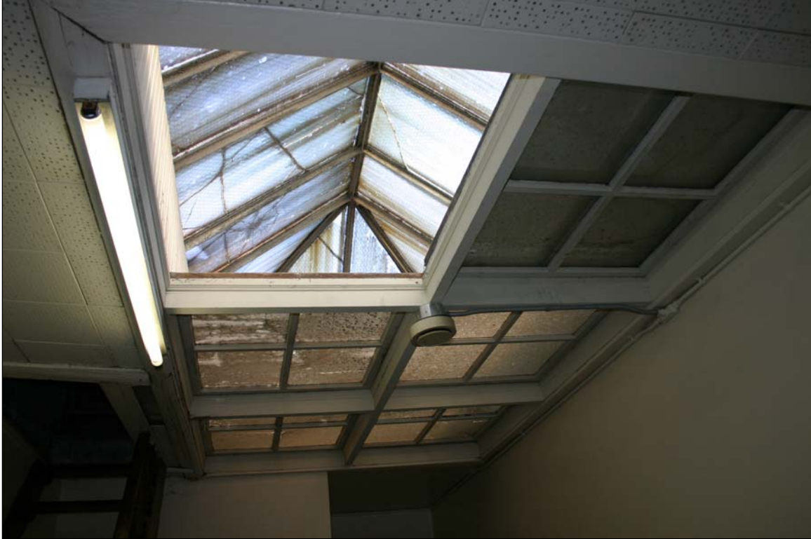
Plate 12 – Staircase skylight, 2005. ( M. Peterson, 2005. )
