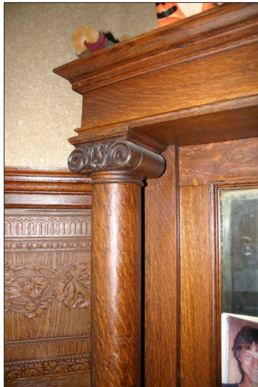
Plate 10 – Detail of woodwork around fireplace, third-floor suite, 2005. ( M. Peterson, 2005. )
