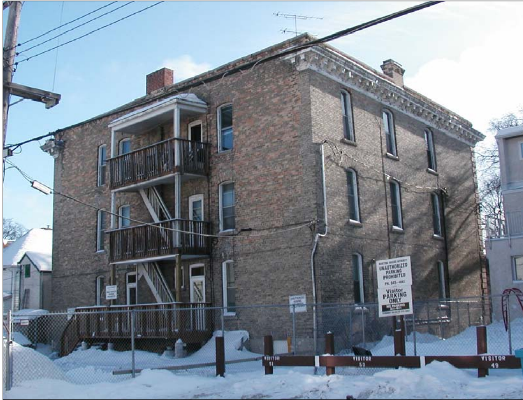
Plate 3 – Rear (north) and west side, 2005. ( M. Peterson, 2005. )
