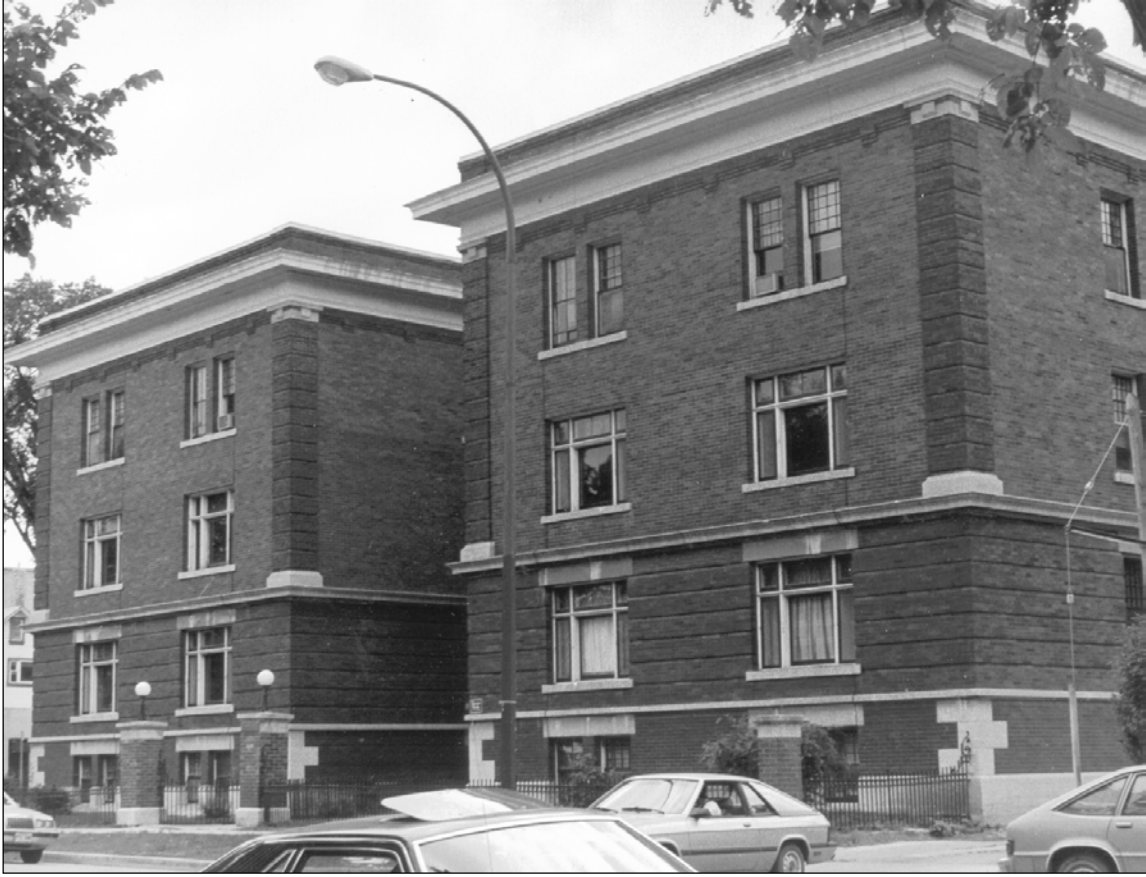
Plate 1 – Congress Apartments, 300 River Avenue, front (north) façade. (M. Peterson, 1989.)
