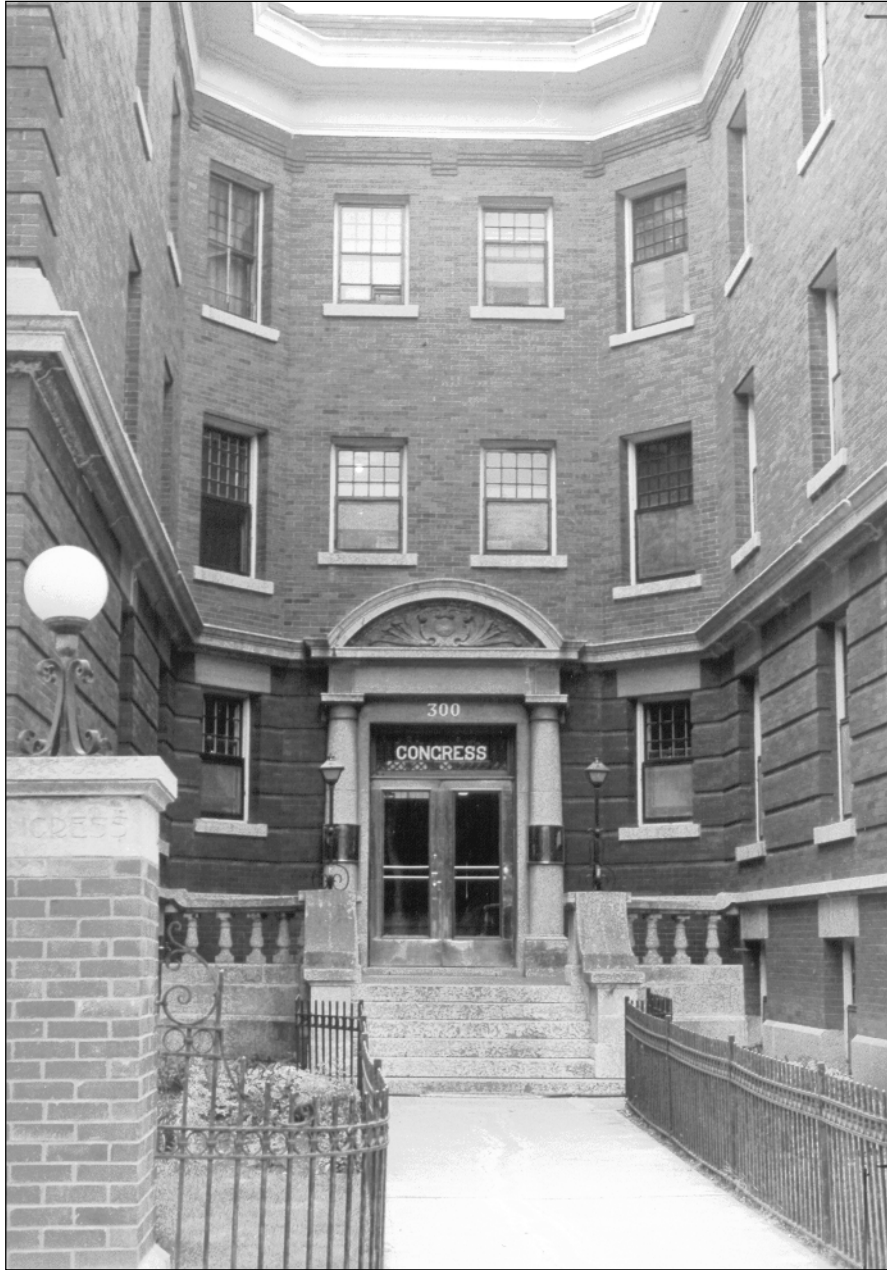
Plate 2 – Congress Apartments, main (north) entrance. (M. Peterson, 1989.)
