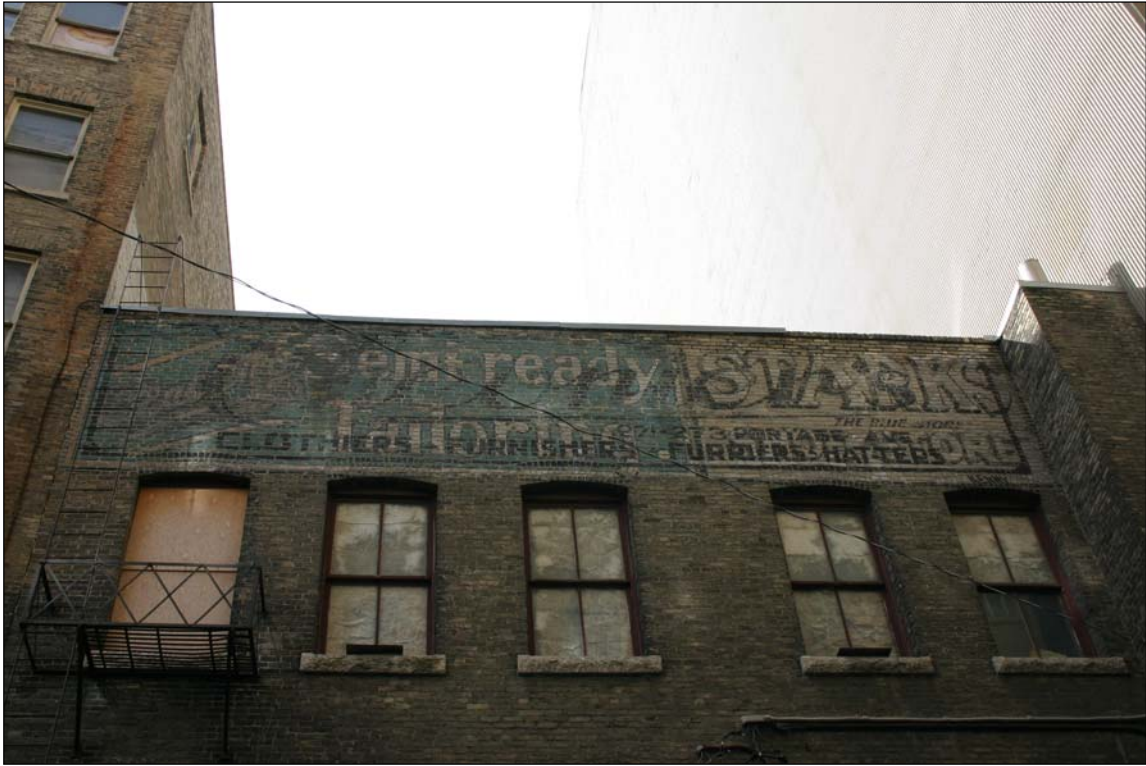
Plate 8 – Signage on rear (north) façade. ( M. Peterson, 2005. )
