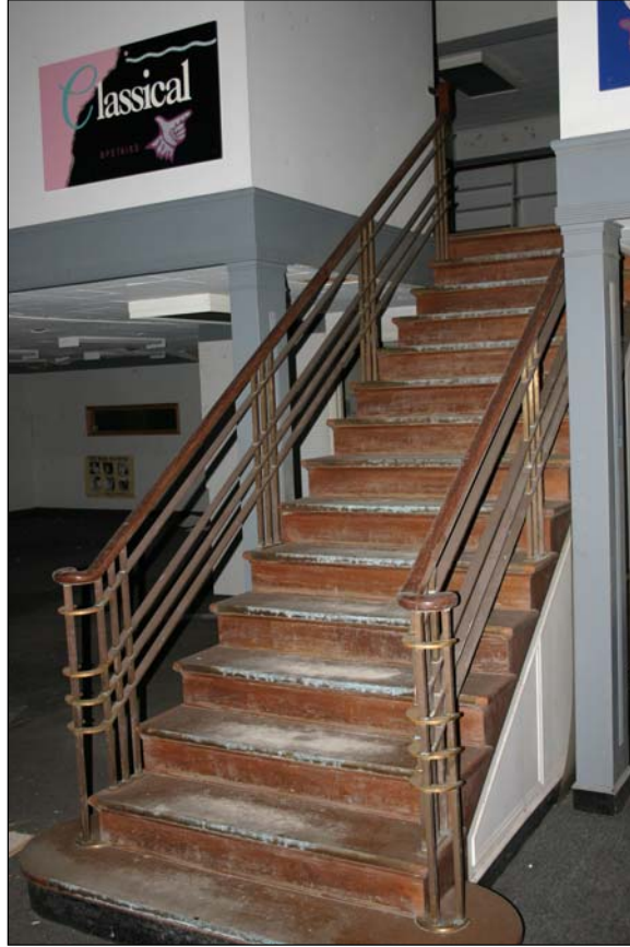
Plate 9 – Mezzanine staircase. ( M. Peterson, 2005. )
