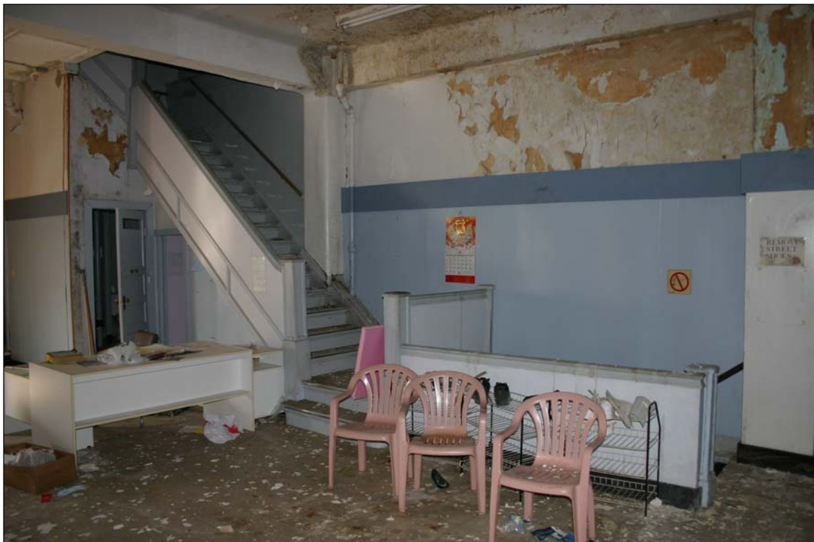
Plate 12 – Second floor staircases. (M. Peterson, 2005.)
