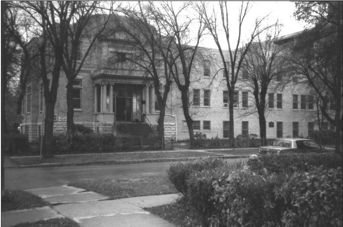
Plate 1 – 210 Rue Masson, front façade. ( City of Winnipeg, 1988. )
