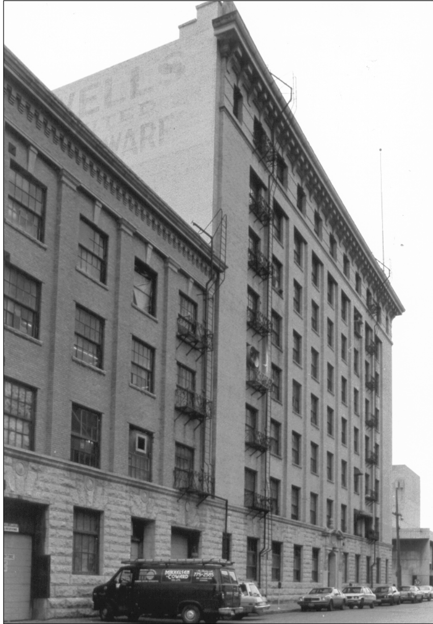
Plate 3 – 136 Market Avenue, north (Market Avenue) façade, 1987. (City of Winnipeg, Planning Department.)
