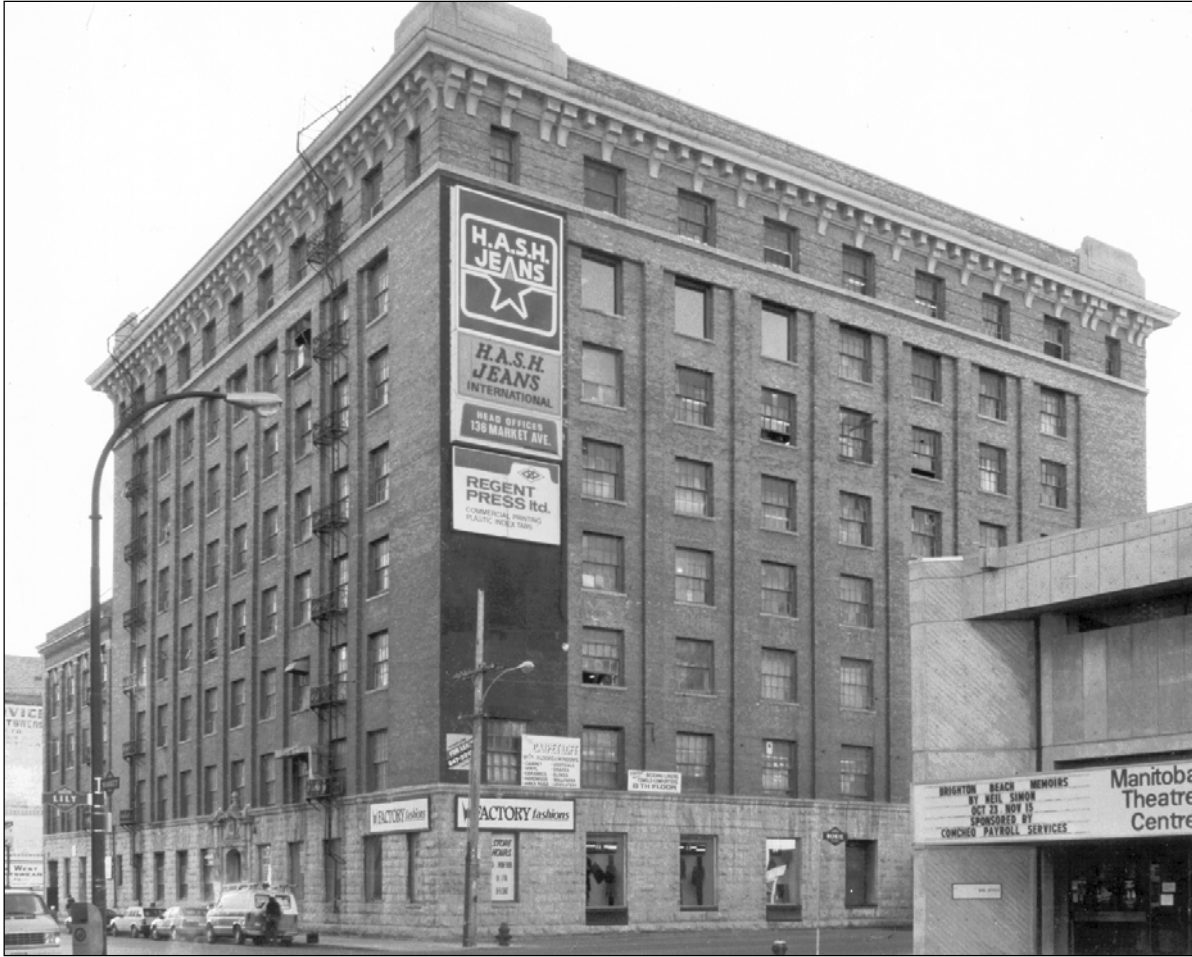
Plate 1 – 136 Market Avenue, Marshall-Wells Hardware Warehouse, 1987. (City of Winnipeg, Planning Department.)
