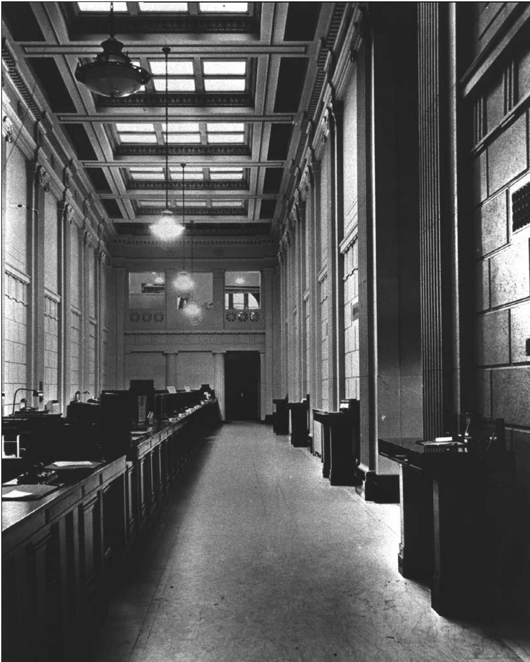
Plate 4 – Interior of Annex, no date. (City of Winnipeg, R. Van Vliet)
