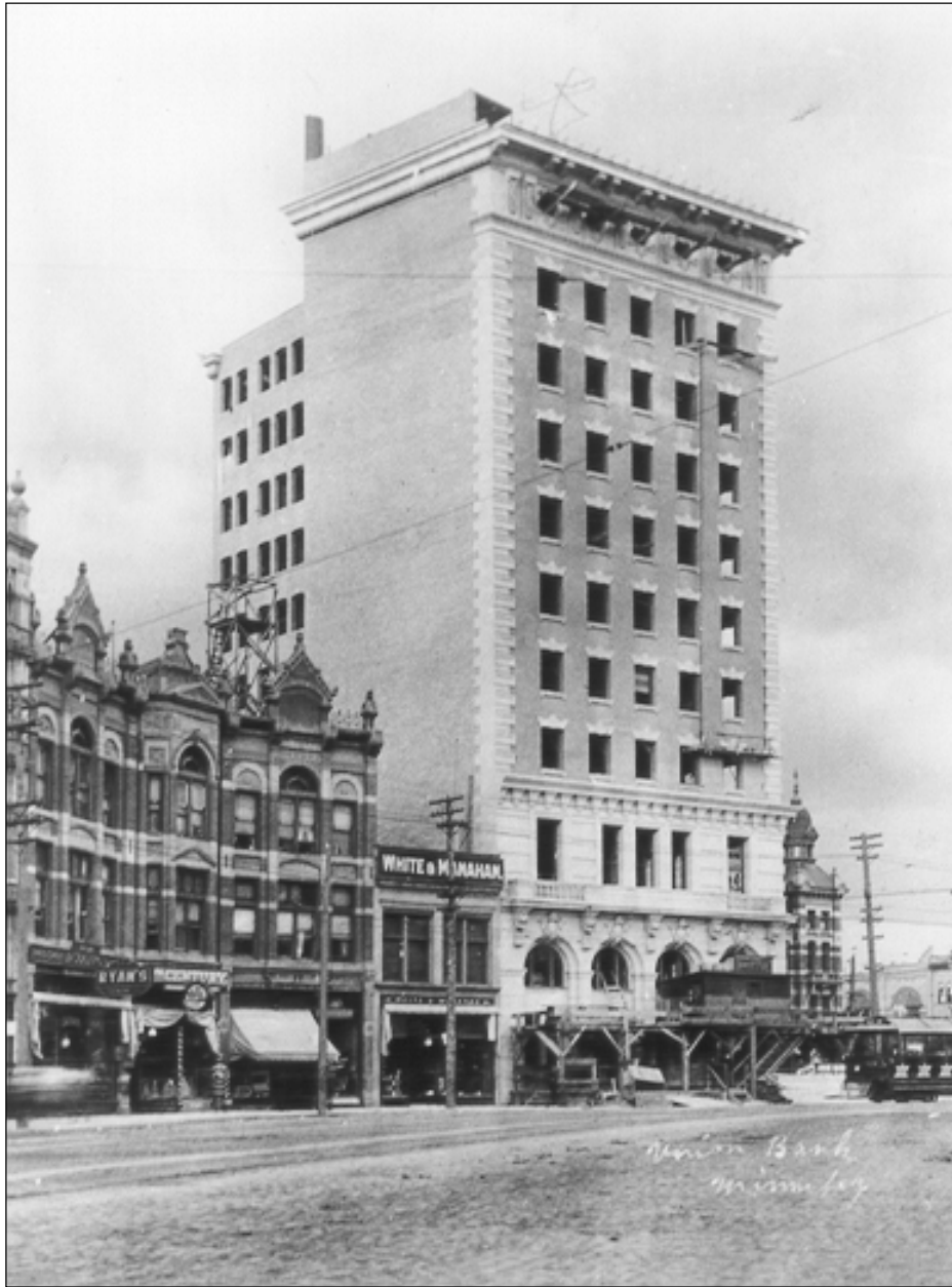
Plate 1 – Union Tower nearing completion, 1904. Note the White and Manahan Store immediately south of the bank. (Courtesy of the Provincial Archives of Manitoba, N1485.)
