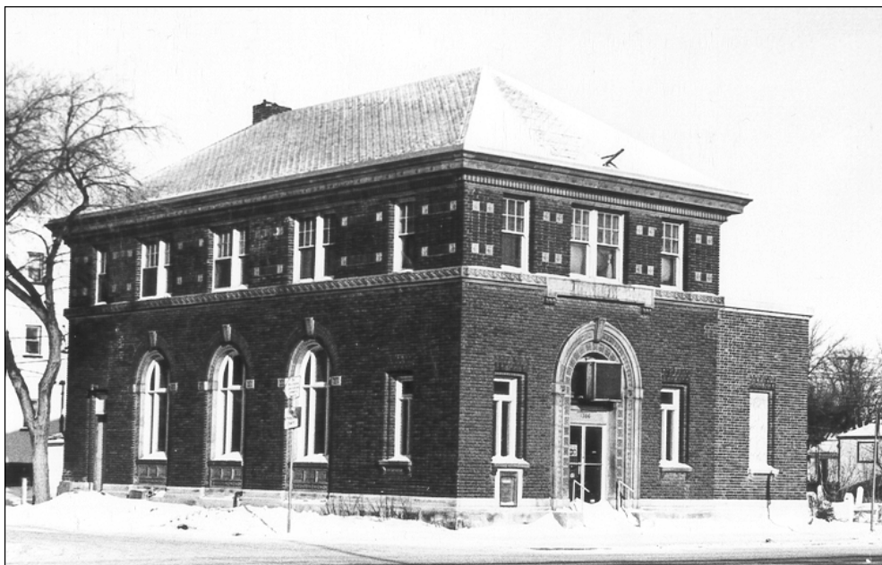
Plate 2 – Merchants’ Bank, front (east) and south façades, no date. (City of Winnipeg, Planning.)
