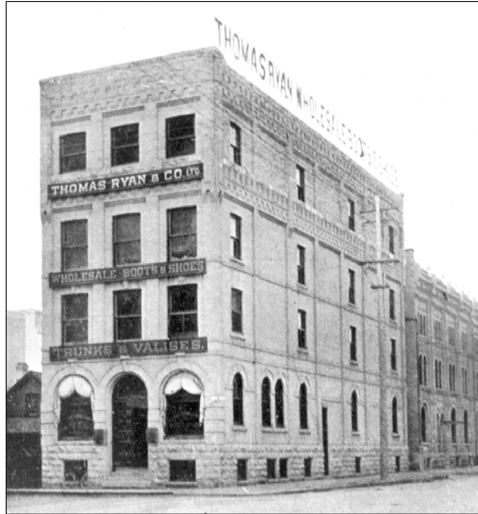
Plate 3 – Ryan Block with a fourth floor, ca.1903. (Courtesy of the Provincial Archives of Manitoba, N1578.)
