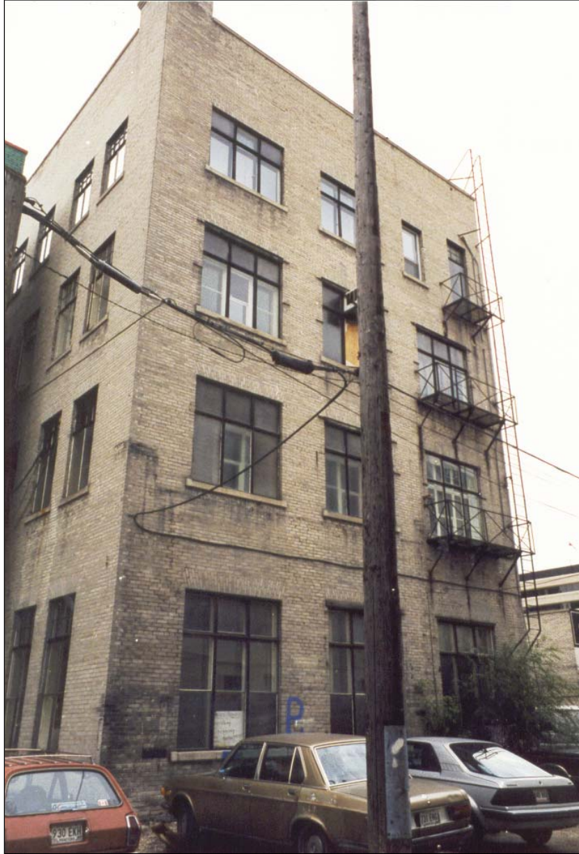
Plate 2 – Garry Block, rear (west) façade, ca.1990. ( City of Winnipeg, Planning Department. )
