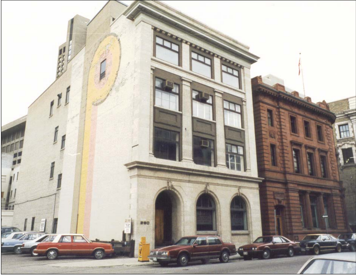
Plate 1 – Garry Block, 290 Garry Street, front (east) façade, ca.1990. Beside is the Comcheq Building (formerly the Canada Permanent Building, 296-98 Garry Street, built in 1909). ( City of Winnipeg, Planning Department. )
