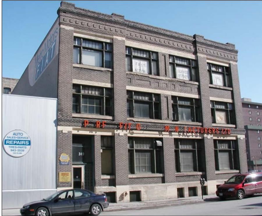
Plate 2 – 319 Elgin Street, Scott Fruit Company Warehouse, front (south) façade, 2004. ( M. Peterson, 2004. )
