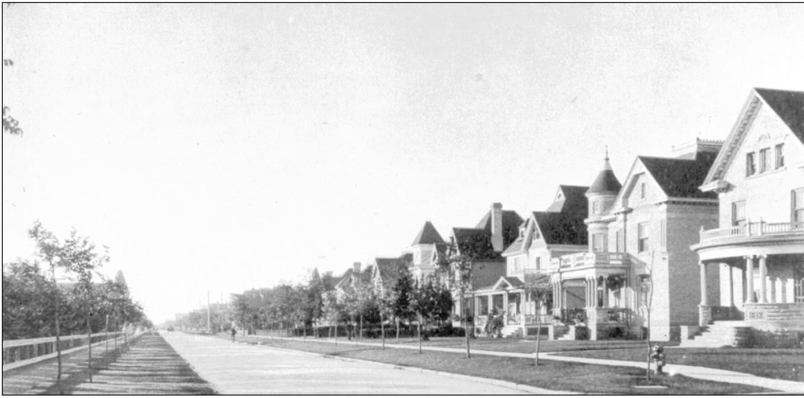
Plate 3 – Edmonton Street, ca.1905. (Courtesy of the Provincial Archives of Manitoba, N9028.)
