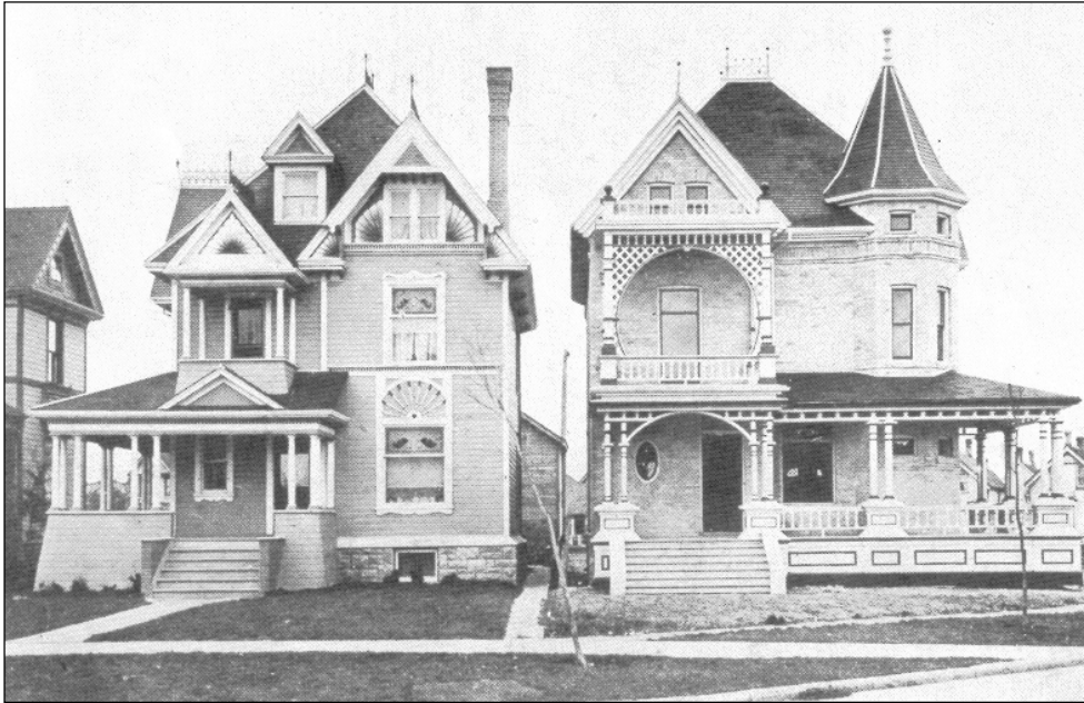
Plate 1 – 454 Edmonton Street, the residence of Hermisdas and Louisa Benard, and its neighbour on the left, cA.1904. A front walk has not yet been added to the Benard house, nor has the lawn been seeded. (Courtesy of the Povincial Archives of Manitoba, N9027.)
