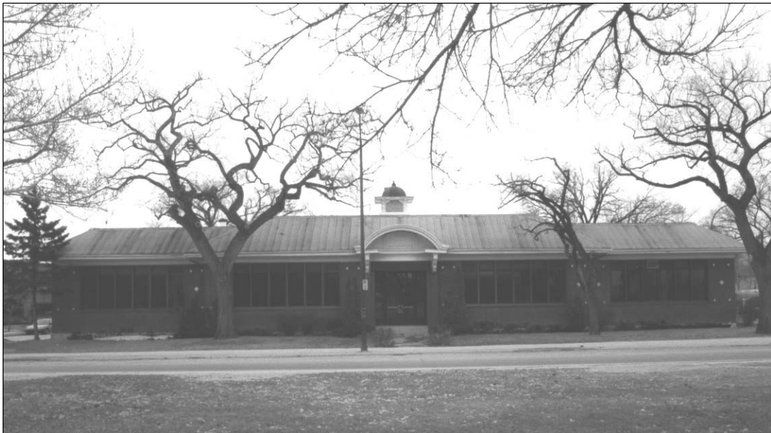
Plate 4 – Former Anna Gibson School, 77 Henderson Highway, front or west façade; built 1919, J.B. Mitchell, architect, Sutherland Construction, general contractor. ( M. Peterson, 1996. )
