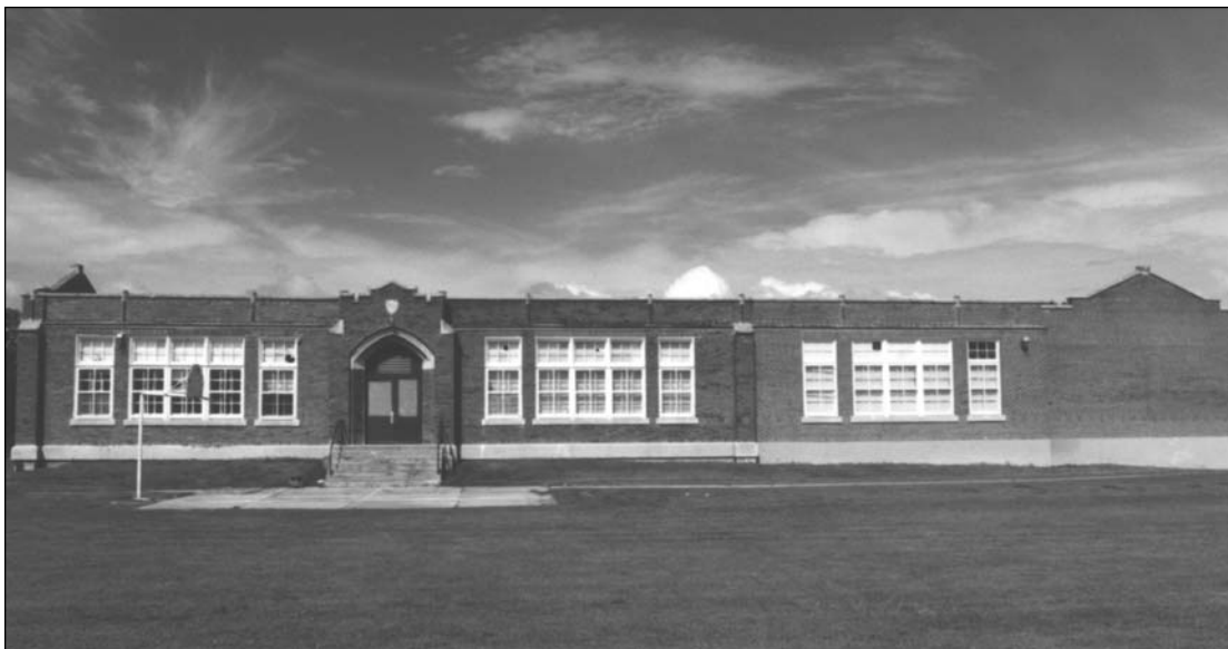
Plate 2 – Sir John Franklin School, 386 Beaverbrook Street, rear or east façade (DEMOLISHED); built 1921, Colonel J.N. Semmens, architect, Fraser and McDonald, general contractors. ( M. Peterson, 1991. )
