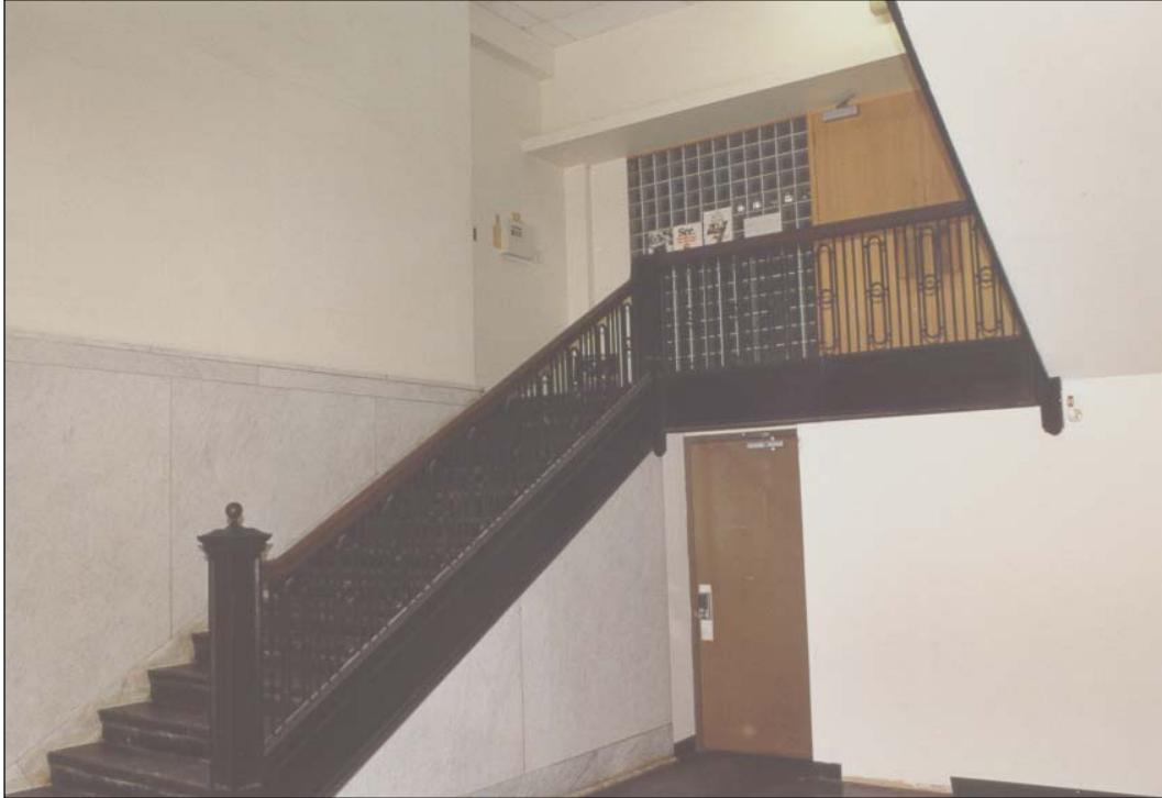
Plate 6 – 365 Bannatyne Avenue, interior staircase. ( M. Peterson, 1992. )
