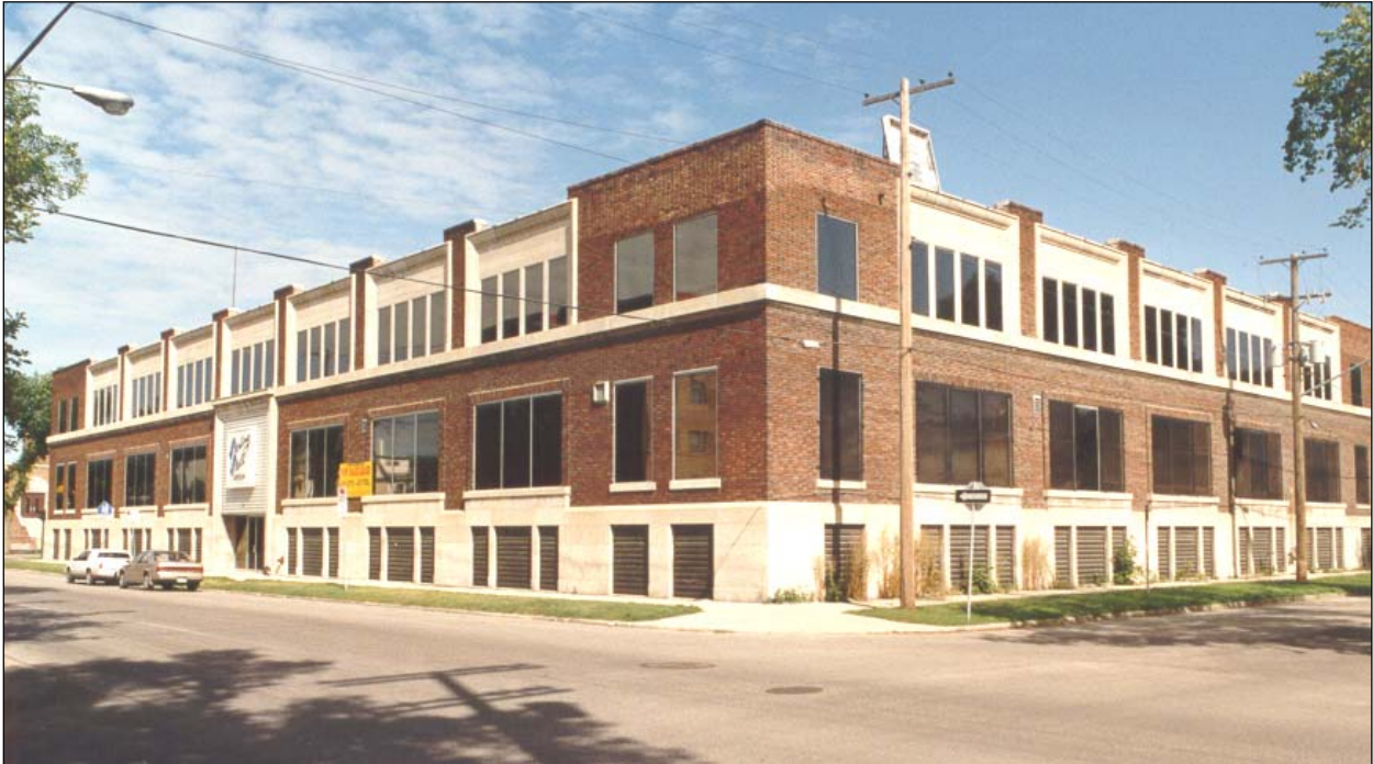
Plate 3 – 365 Bannatyne Avenue, south and east façades. ( M. Peterson, 1992. )
