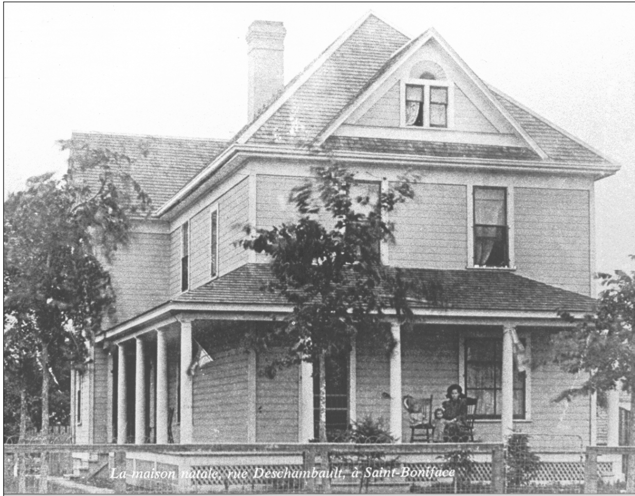
Plate 3 – 375 Rue Deschambault, Roy House, ca,1915 (built ca.1905). (Courtesy of the City of Winnipeg, Planning Department.)
