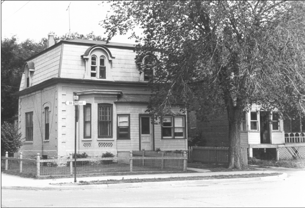
Plate 1 – 453 Qu'Appelle Avenue, Kerr House, 1969. ( Courtesy of the Provincial Archives of Manitoba, Architectural Survey. )
