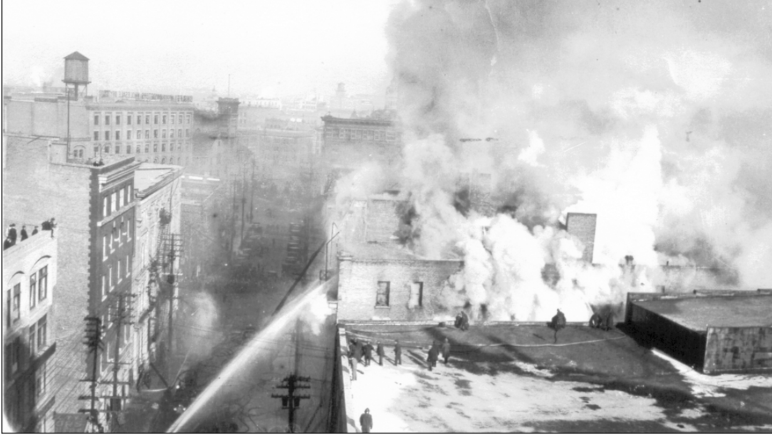
Plate 1 – A fire in the Hammond Building on October 31, 1923, which gutted most of the interior. (Courtesy of the Provincial Archives of Manitoba Photograph Collection.)
