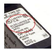
Sample Labels on Combination-Type AFCI Breakers
