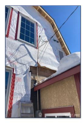
Where alterations to buildings create interference with an existing energized electrical service, Code minimums and safety must be maintained. Where that is not possible due to the complexities of construction, a temporary service will be required.
