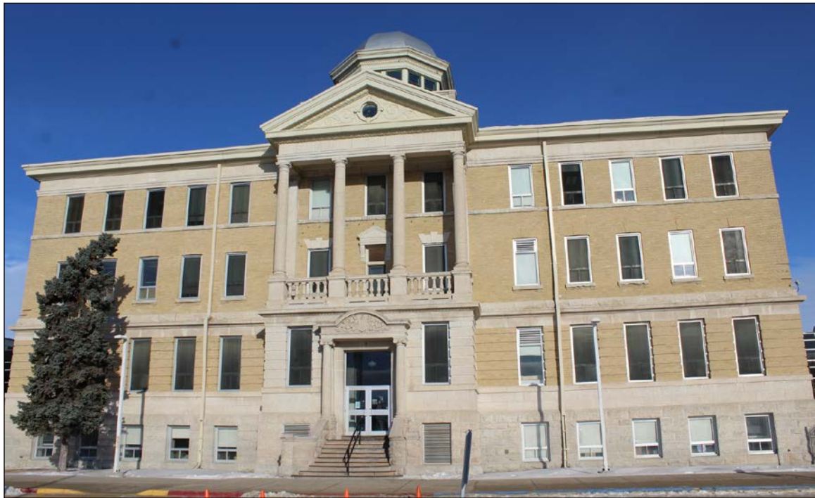
Plate 7 – Administration Building, Manitoba Agricultural College, 139 Tuxedo Avenue, 2018. ( M. Peterson, 2018. )
