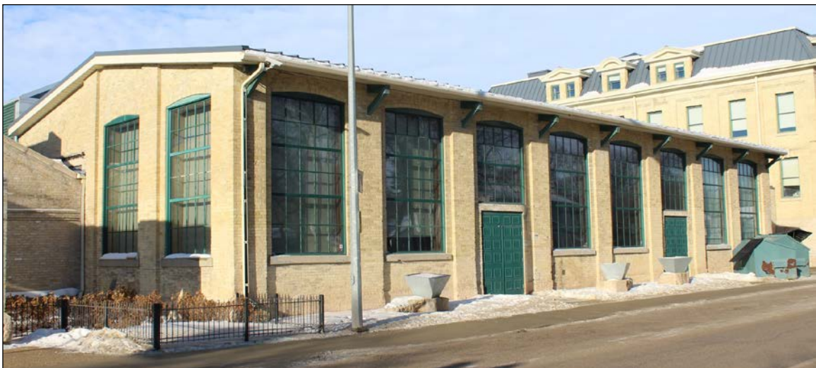
Plate 25 – Power House (1921 section), Manitoba Agricultural College, 139 Tuxedo Avenue, south and east façades, 2016. (M. Peterson, 2016.)
