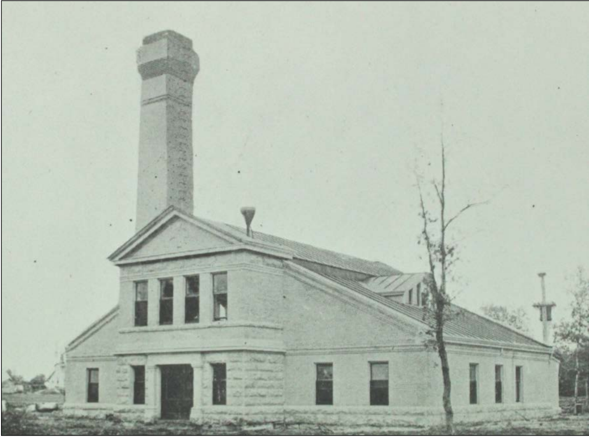
Plate 31 – Power House, Manitoba Agricultural College, 139 Tuxedo Avenue, 1906. ( Archives of Manitoba, Manitoba Agricultural College-Tuxedo Site 12, N8687. )
