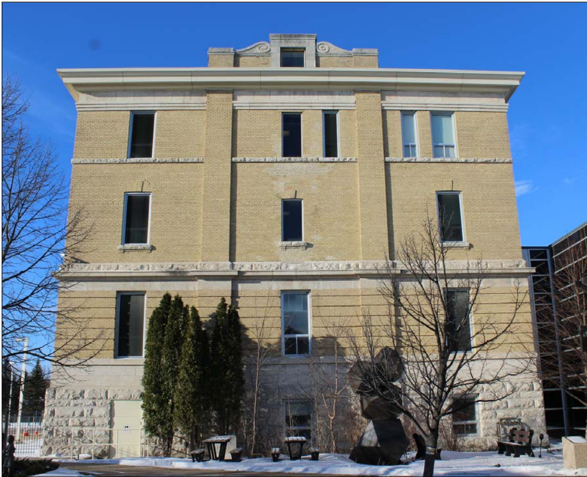
Plate 21 – Administration Building, Manitoba Agricultural College, 139 Tuxedo Avenue, east façade, 2018. (M. Peterson, 2018.)
