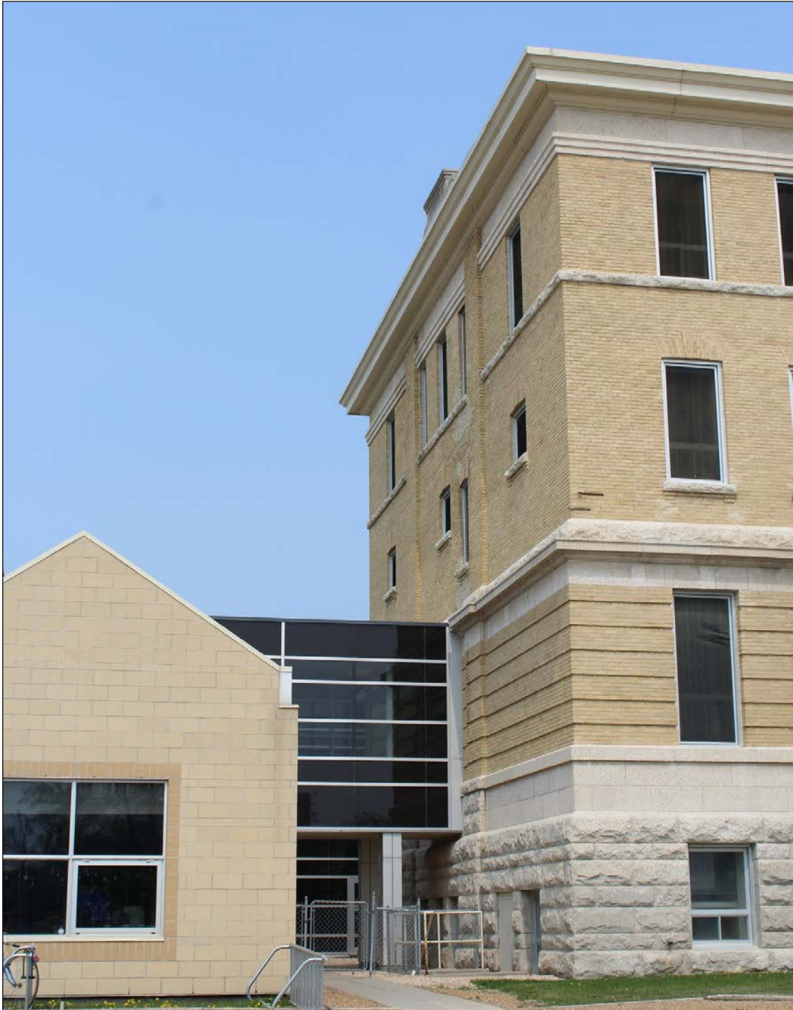
Plate 20 – Administration Building, Manitoba Agricultural College, 139 Tuxedo Avenue, west façade, 2016. (M. Peterson, 2016.)
