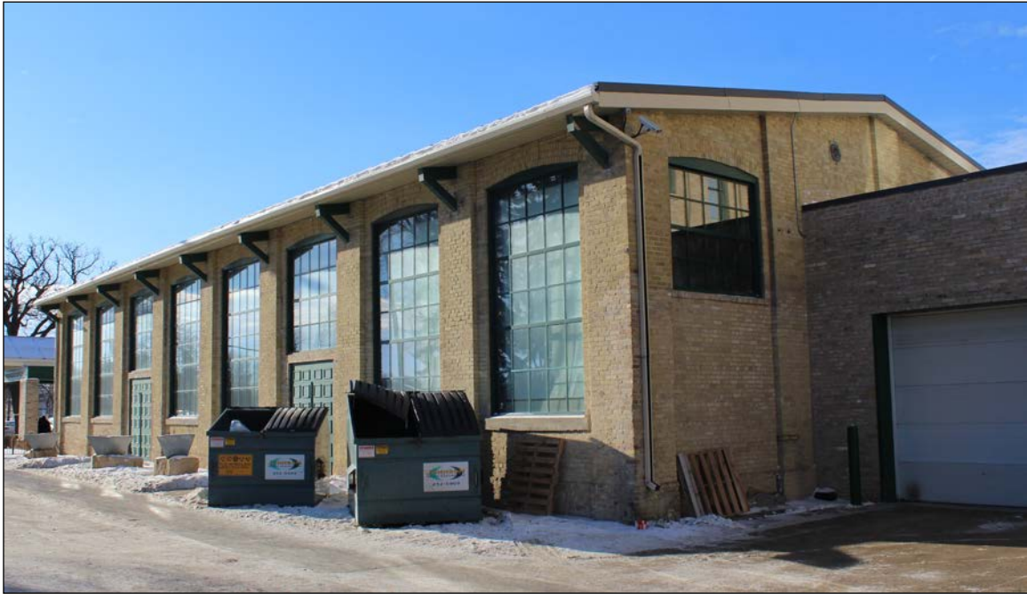
Plate 26 – Power House (1921 section), Manitoba Agricultural College, 139 Tuxedo Avenue, north and east façades, 2018. (M. Peterson, 2018.)
