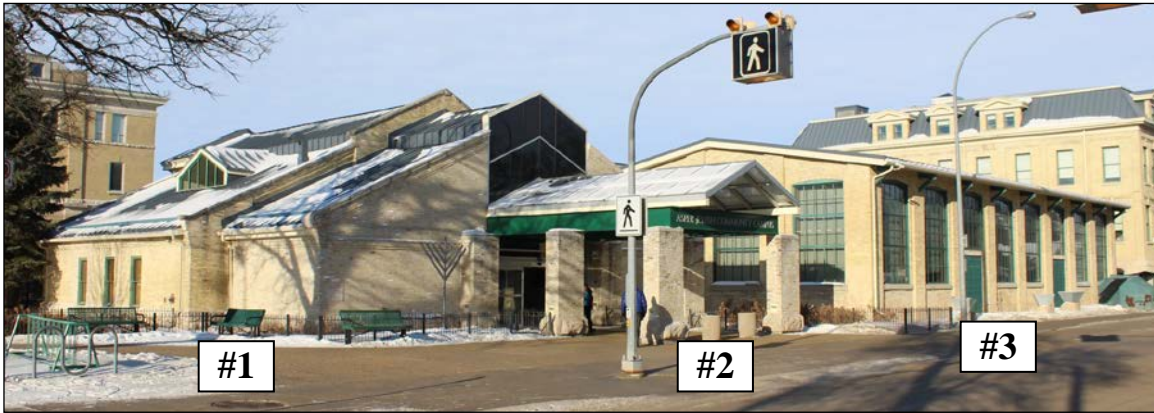
Plate 8 – Power House, Manitoba Agricultural College, 139 Tuxedo Avenue, 2018. Pictured are the original building, 1906 (#1), 1997 entrance (#2) and 1921 addition (#3). ( M. Peterson, 2018. )
