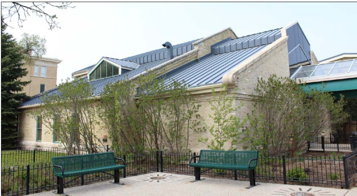
Plate 23 – Power House (1906 section), Manitoba Agricultural College, 139 Tuxedo Avenue, rear (east) and south façades, 2016. (M. Peterson, 2016.)
