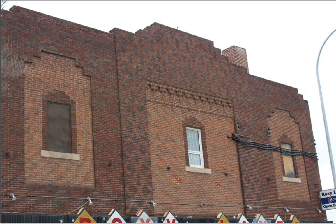
Plate 11 – Roxy Theatre, 385 Henderson Highway, detail of front (west) façade, 2022. ( M. Peterson, 2022. )
