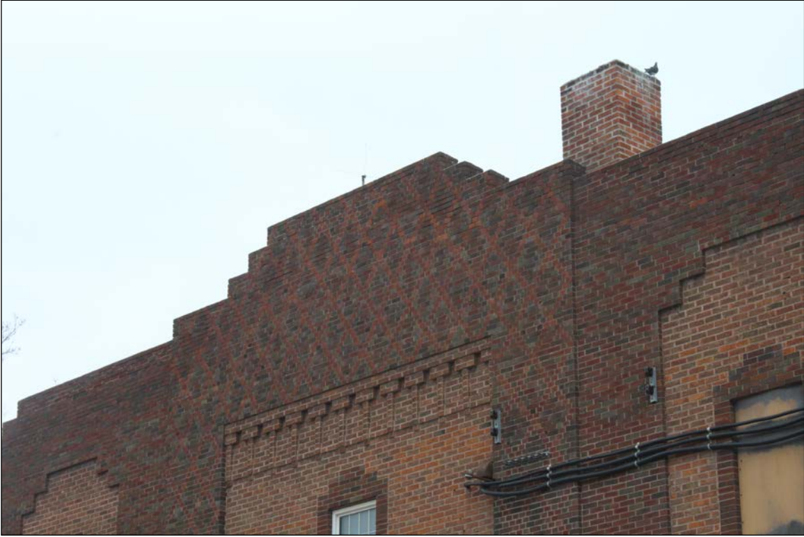
Plate 12 – Roxy Theatre, 385 Henderson Highway, detail of front (west) façade, 2022. ( M. Peterson, 2022. )
