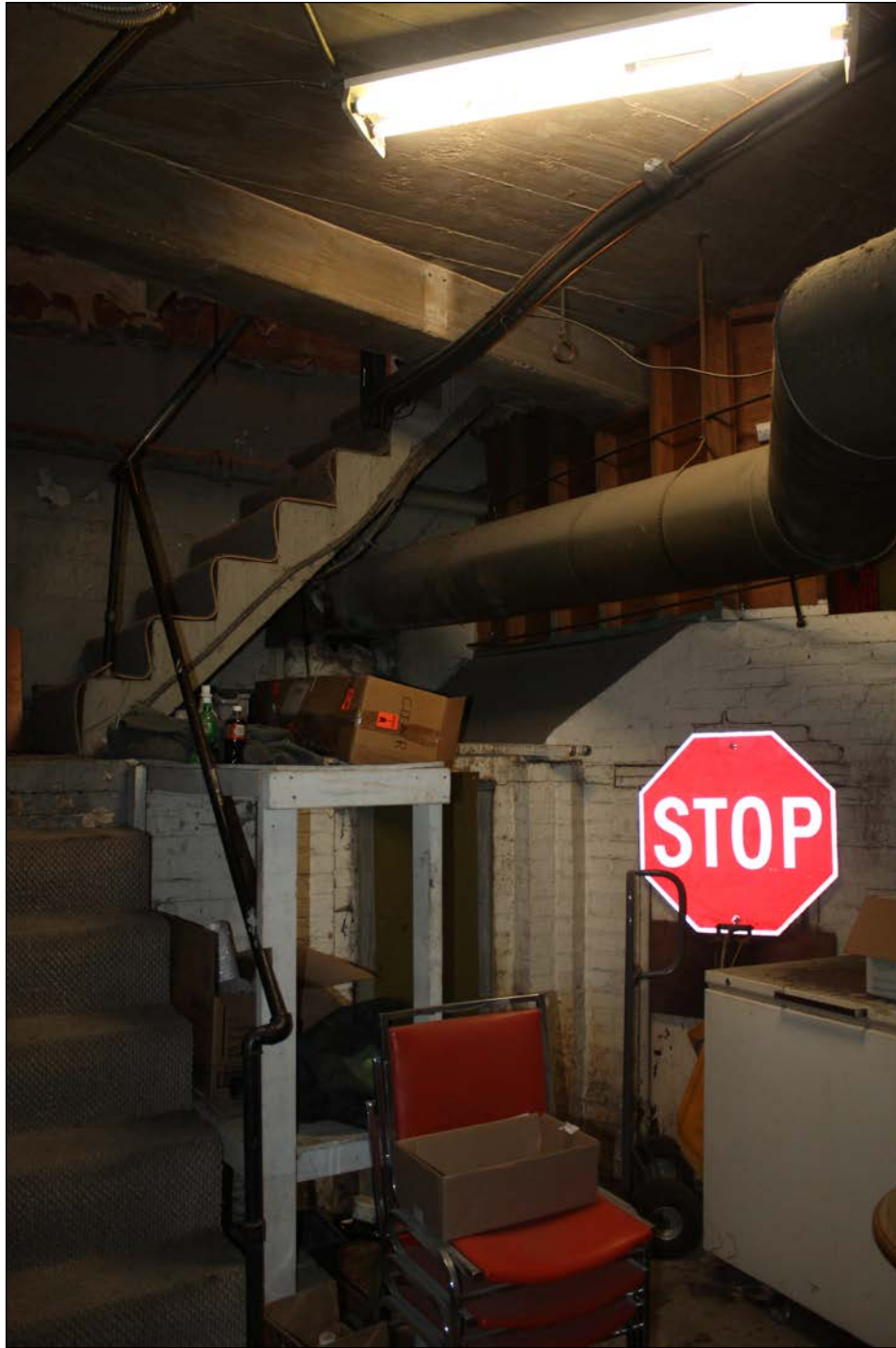
Plate 16 – Roxy Theatre, 385 Henderson Highway, basement stairs, 2022. (M. Peterson, 2022.)
