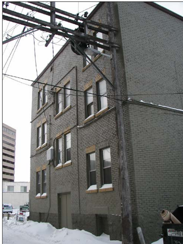
Plate 9 – Windsor Hotel, 187 Garry Street, rear (east) façade. (M. Peterson, 2005.)
