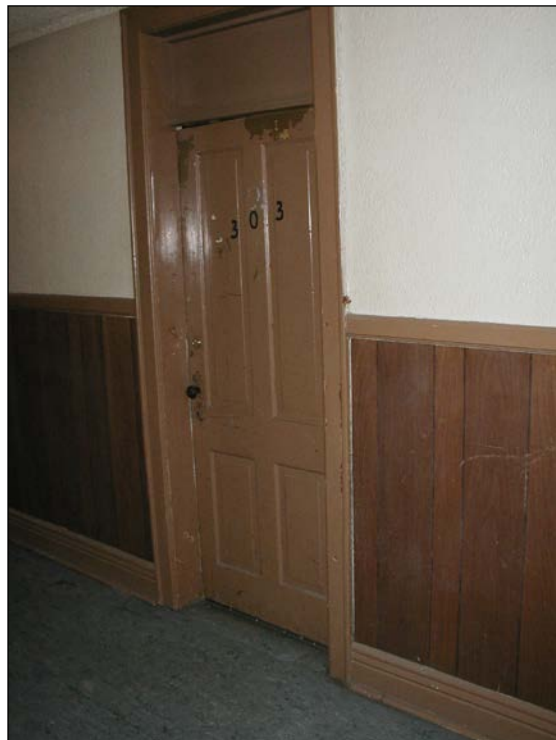
Plate 17 – Windsor Hotel, 187 Garry Street, original door, third floor. ( M. Peterson, 2005. )
