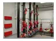
The sprinkler system is a wet system which covers the whole building. The main control valve is in the basement mechanical room.
