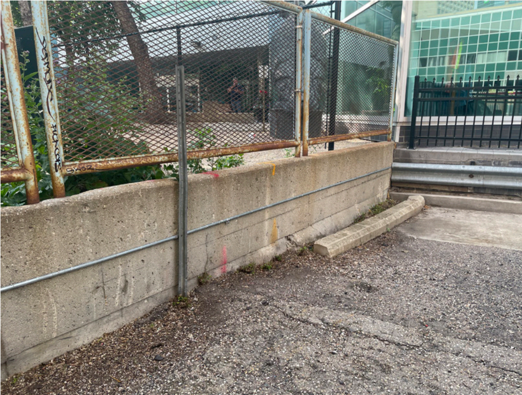
View of northeast retaining wall (from alley) July 2023
