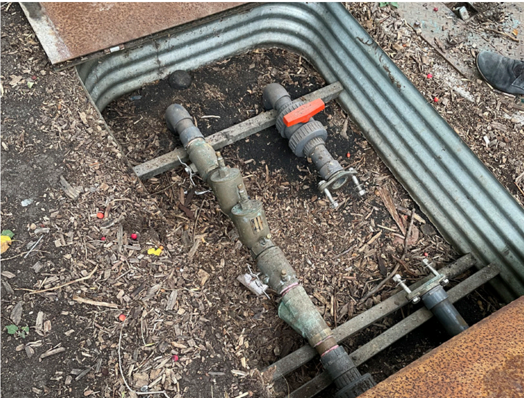
View of abandoned water meter pit September 2023
