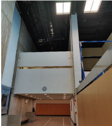
Photo 4: Proposed Mezzanine Area For F-2 & F-4 (Above Existing Office Space)
