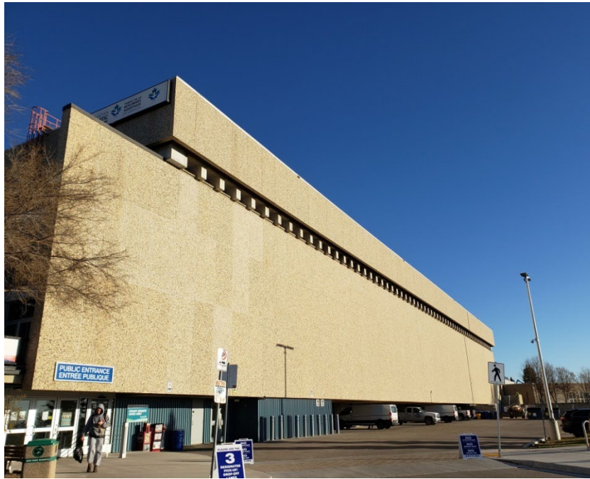
Photo 1: Main Pool Area South Wall
