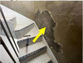
Delamination was also observed on the sides of the north 3 metre springboard platform (Photographs 3.2.3.4-4). Localized repairs are recommended.
