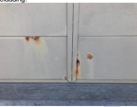
Photograph 3.3.1.13-5: Typical example of delaminating coating observed on horizontal metal cladding.
