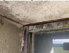
Photograph 3.3.1.6-6: Example of localised damage of a pre-cast concrete feature at jambs/between window bays exhibiting localized deterioration, cracking and spalling.
