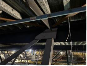
The suspended ceiling panels over the main pool are suspend from the steel roof deck. The support cables and roof framing appeared to be in good condition.
