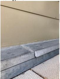
Photograph 3.3.1.13-8: View of sealant repair completed at curb next to entrance.
