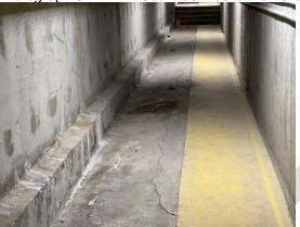
Photograph 3.2.1.2-2: North service tunnel. Cracking heaving and delamination of floor slab visible.
