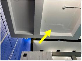
Photograph 3.2.3.4-3: Delamination on internal stairwell walls.
