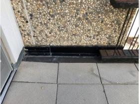
Recommendation 3.3.1.1-1: It is recommended that the cause of the pre-cast panel displacement be investigated further to assess the condition of the underlying anchorage. We recommend investigating the panels located above the main pool entrance on the south elevation as a starting point. The scale of the investigation, including access and selective demolition is outside the scope of this report.
