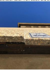
Photograph 3.3.1.1-4: Displacement of panels above the main pool entrance on the south elevation taken from the arial lift and showing vertical displacement as evidenced by torn sealant joint.
