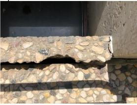
Photograph 3.3.1.6-4: Typical example of degraded and/or missing glazing sealant and sealant beads at frame perimeter to adjacent soffit, pre-cast concrete features at jambs, and pre-cast exposed aggregate sloped sills.
