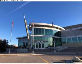
The condition of the cladding on the Aquatic Hall of Fame, coupled with the findings of the Curtainwall Leakage Review by Pinchin dated January 10<sup>th</sup>, 2020, which included selective demolition to review the condition of underlying envelope elements, warrants a comprehensive report on this part of the facility. The following is a summary of our non-destructive visual assessment. Note that no apparent repairs were completed since the issuance of the Pinchin report.
