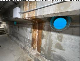
Photograph 3.2.3.1-4: West pool wall showing leakage and delamination.
