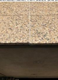
Photograph 3.3.1.1-6: Typical example of localized staining as a result of corrosion of iron ore inclusions in the exposed aggregate. Photo taken on south elevation but condition observed throughout.
