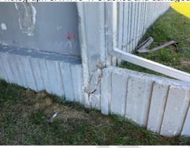
Recommendation 3.1.1.10-1: Repair existing retain wall and install new expansion joint.
