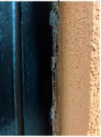
Photograph 3.3.1.8-3: Partial view of east column base showing ice and frost accumulation. Note also ice accumulation at base of wall.
