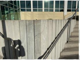
Recommendation 3.1.1.4-1: Localized concrete repairs are required in the short term and will consist of removing the loose concrete down to a sound substrate, preparation of the substrate and infilling with a proprietary repair material or ready-mix concrete.
