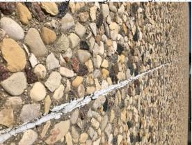
Photograph 3.3.1.1-10: Base of wall transitions from pre-cast panel to flashing at with wing walls adjacent the entrance on the west elevation were found to be severely degraded. Entrance on south side of Aquatic Hall of Fame shown.
