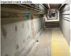
Photograph 3.2.3.1-2: North tank wall looking west from east end.
