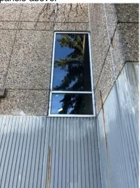
Photograph 3.3.1.10-3: Typical example of vertical sealant joint in pre-cast fluted concrete panel.
