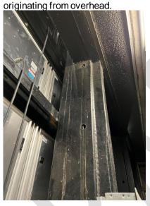
Photograph 3.3.1.14-2: View of water staining observed on back side of scoreboard, originating from overhead.
