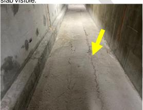
Photograph 3.2.1.2-3: Delamination of floor slab.
