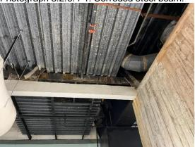
Recommendation 3.2.6.4-1: Clean and paint corroded steel beam.
