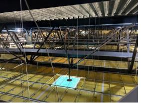
.2 Catwalks are typically located within the centre of each triangular roof truss in the north-south direction and are connected to two main catwalks that run in the east-west direction
