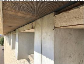
Photograph 3.3.1.6-2: Typical example of stucco clad soffits showing displacement from underlying wood framing, evidence of corrosion of metal corners and lath, and evidence of prior wetting of underlying wood framing.
