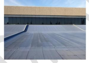
Photograph 3.3.3.1-3: Showing typical buckling in roof cover, east roof facet.
