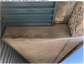
Photograph 3.3.1.7-3: Partial view showing typical condition of stuccoed soffit along north elevation (looking west) showing typical example of localized patch repair/painting and stains.
