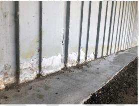
Photograph 3.3.1.4-4: Typical example of water staining and rust marks originating from within the mesh soffit, appeared to align with mechanical exhaust ducts. Photo taken on south elevation.
