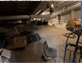
Photograph 3.2.2.1-5: Crawlspace on west side of the Lap Pool. Discontinuous vapour visible.
