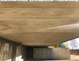
Photograph 3.3.1.7-2: Localized repairs required at the west end of the south soffit, at the underside outside corner where the stucco has cracked and the corner does not appear to be reinforced with mesh.
