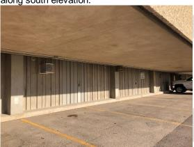
Photograph 3.1.1.9-2: Partial view of cast-in-place 10" thick corrugated concrete wall along north elevation.
