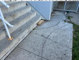
Recommendation 3.1.1.8-1: Seal precast joints with an elastomeric joint sealant. Clean and paint precast connections.
