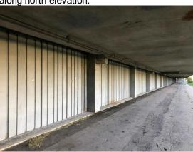
Photograph 3.3.1.4-3: Typical example of delaminating coating and missing sealant at base of wall. Photo taken on north elevation.
