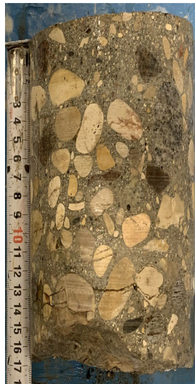
Figure 4 – Core No. 4 (Brock St)
