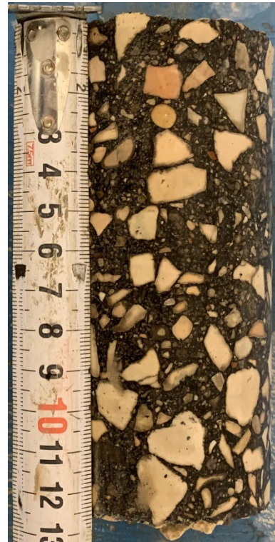
Figure 10 – EB BH-04 (Taylor Ave)
