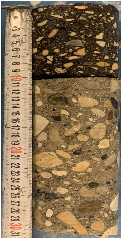
Figure 9 – EB BH-03 (Taylor Ave)
