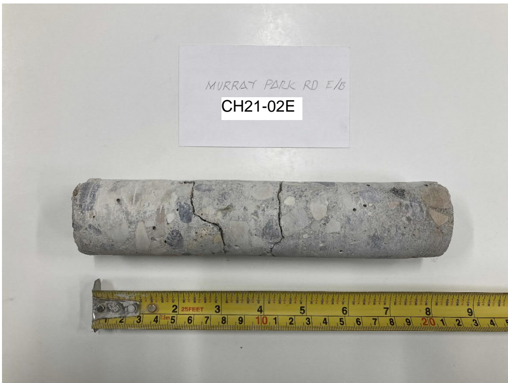
Photograph 6: CH21-02E - Murray Park EB (Cree Crescent to Saulteaux Crescent)
