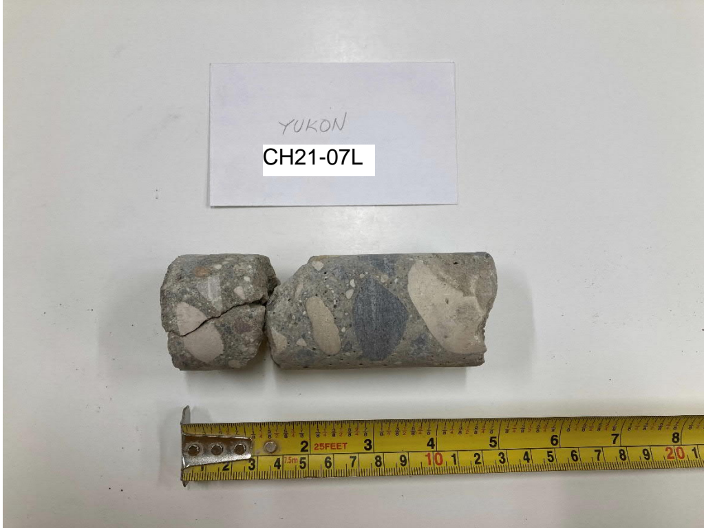
Photograph 27: CH21-07L - Yukon Avenue (St. James Street to Milt Stegall Drive)
