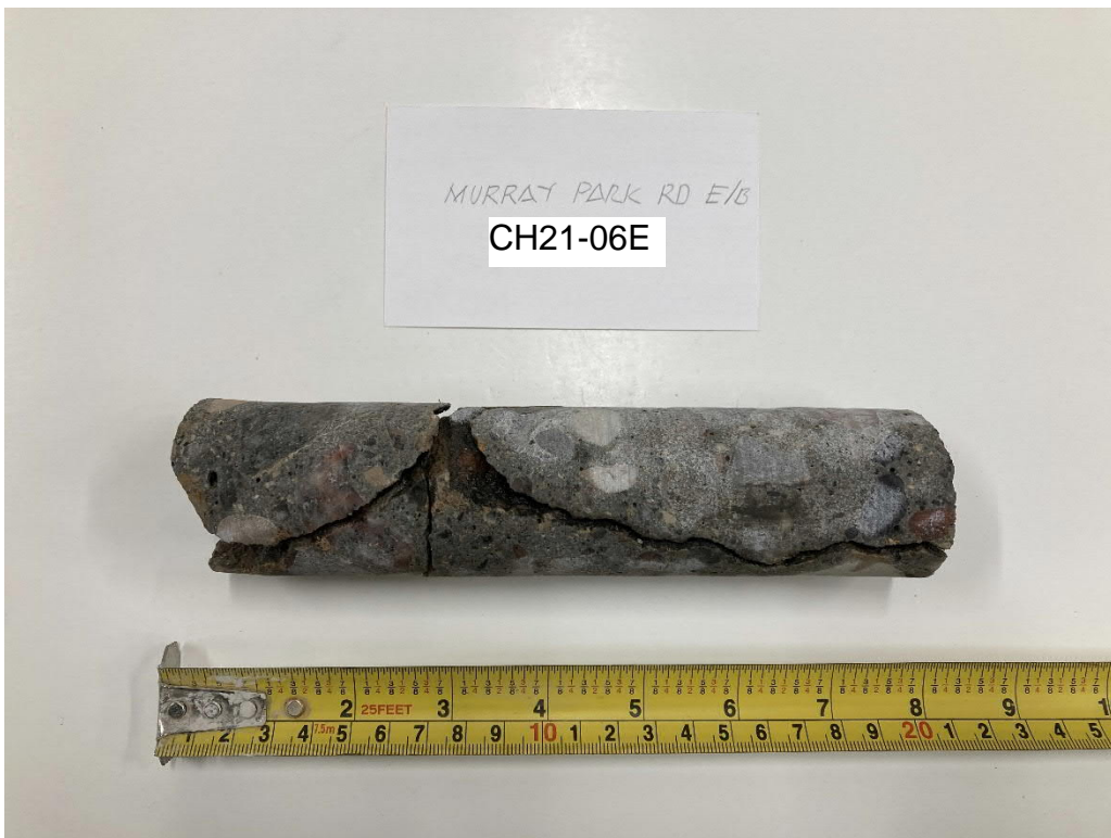
Photograph 10: CH21-06E - Murray Park EB (Cree Crescent to Sauleaux Crescent)
