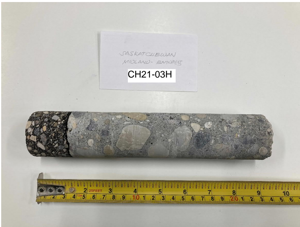
Photograph 16: CH21-03H - Saskatchewan Avenue (Midland Street to Empress Street)
