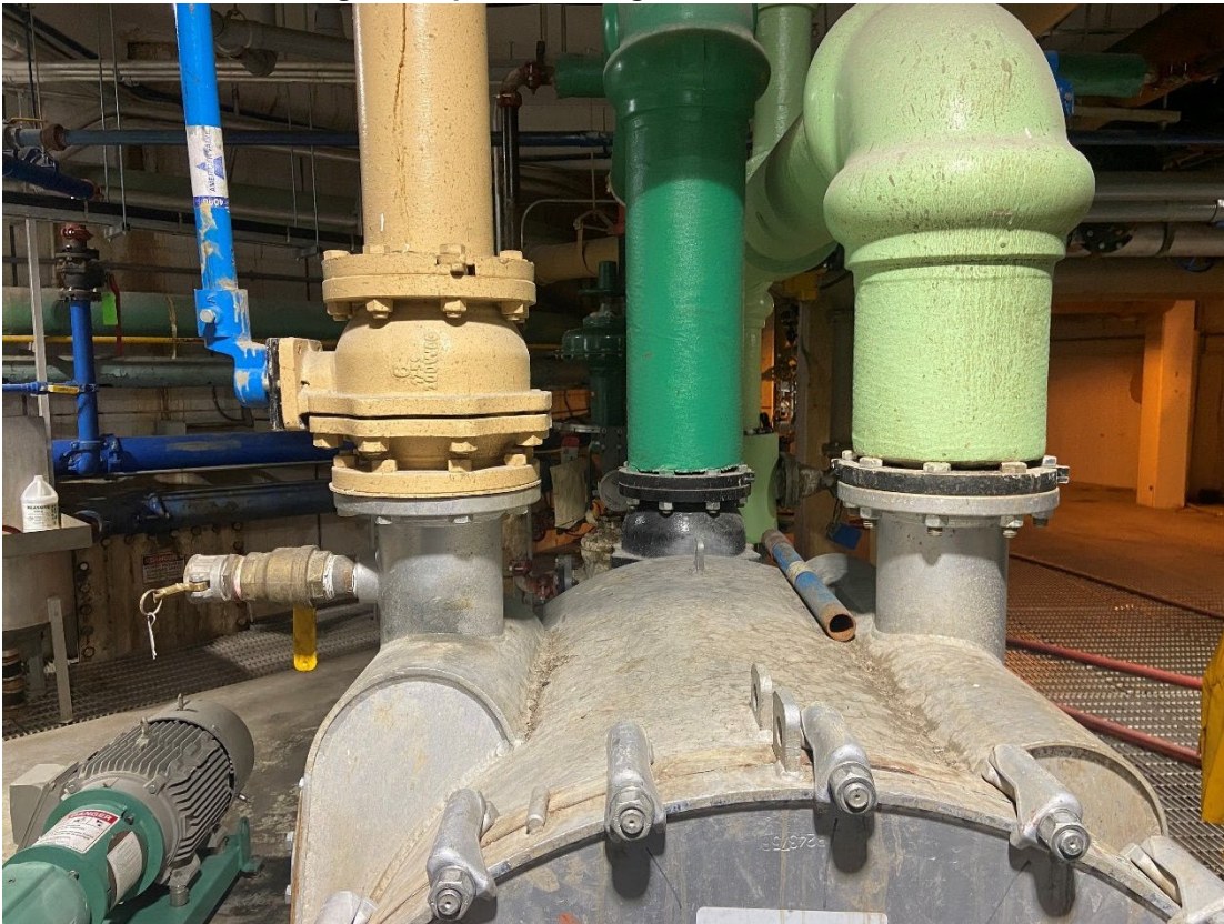
Digester Spiral Exchanger Top Connections
