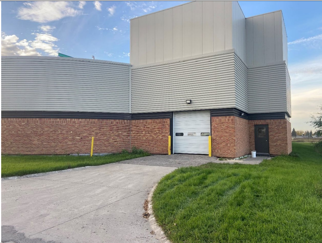
Exchanger Unload Location Outside
