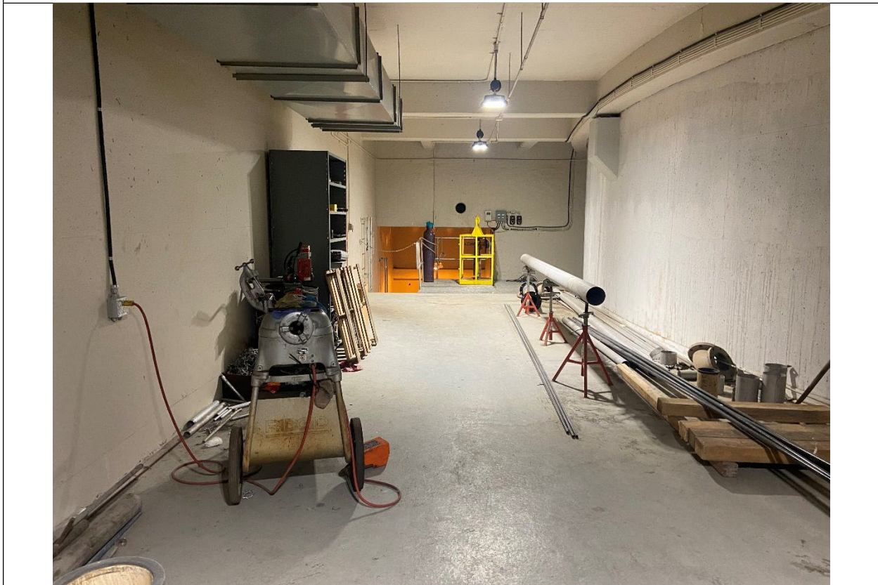
Digester Spiral Exchanger Storage Gallery 2 (4 Exchangers)
