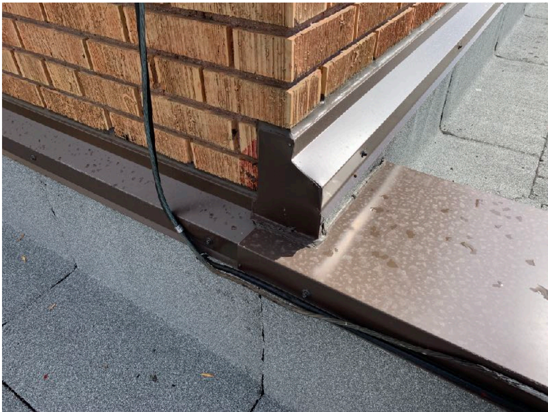
Typical base-bid copings & metal siding.
