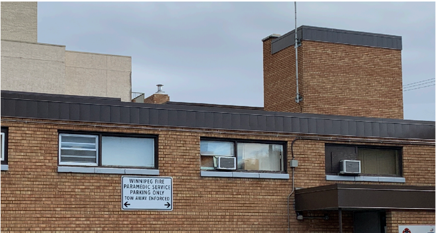
Typical base-bid copings & metal siding.
