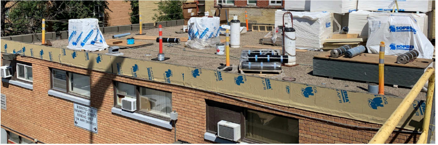
Typical parapet pony wall and membranes.
