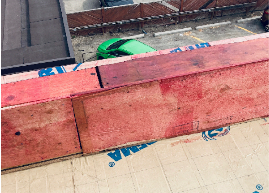
Typical new parapet construction.
