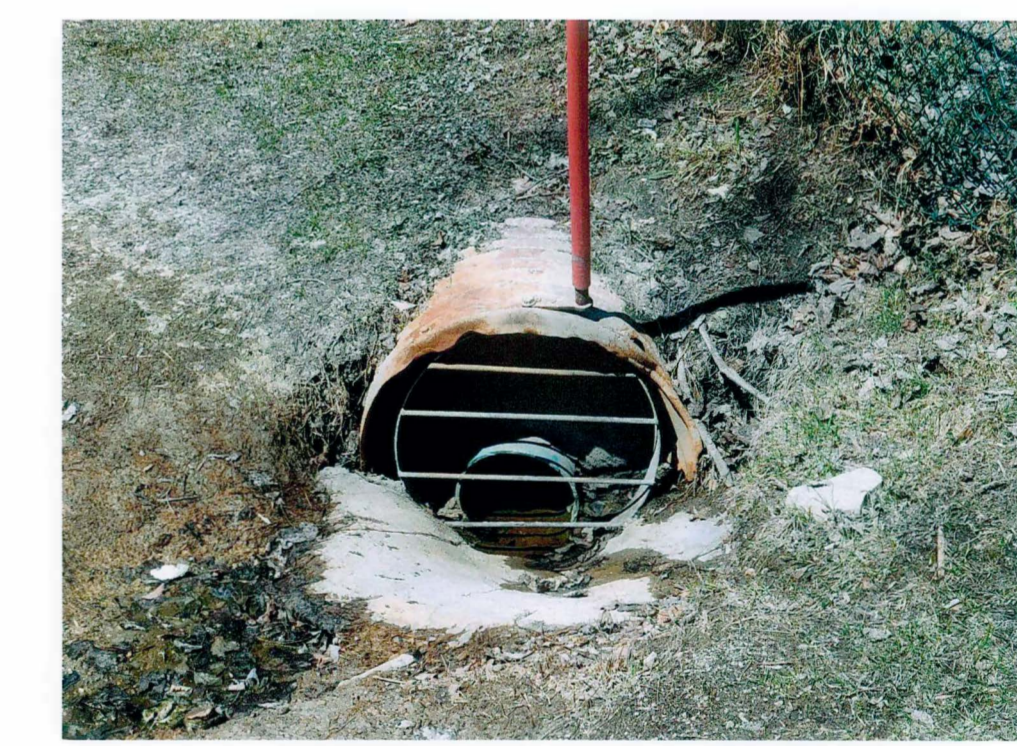
PICTURE 3: CONCRETE FILLED LDS TO BE REMOVED AND DISPOSED OF
