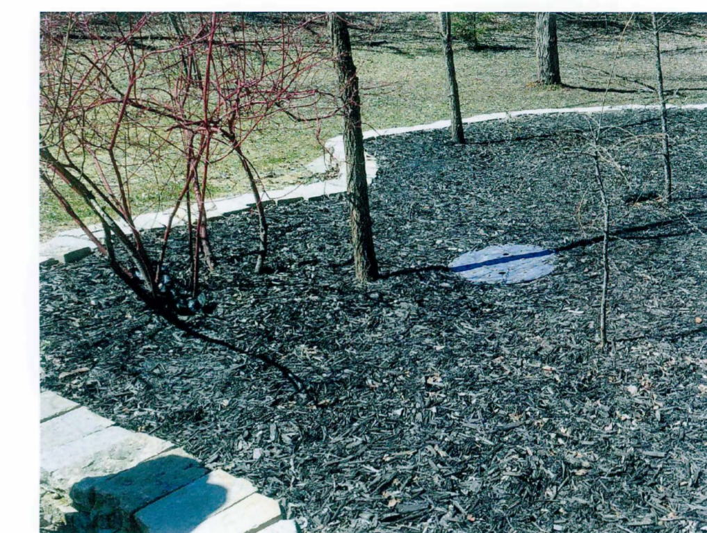
PICTURE 1: EXISTING MANHOLE TO BE ABANDONED
