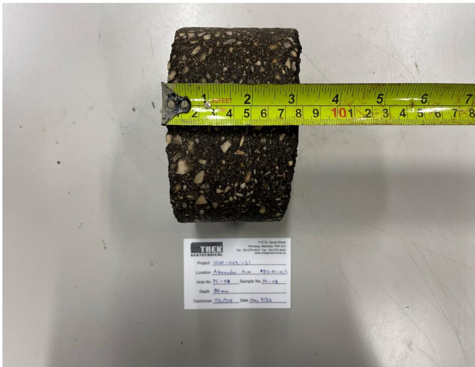
Photo 2: Pavement Core Sample PC-08
