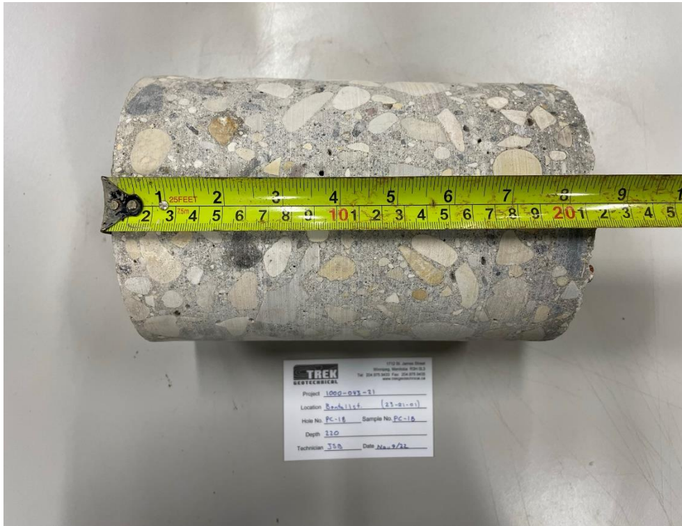
Photo 1: Pavement Core Sample PC-18
