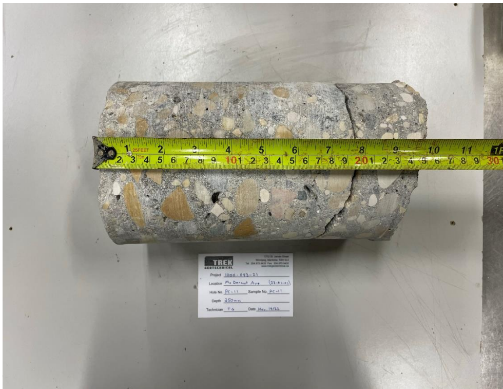
Photo 2: Pavement Core Sample PC-11
