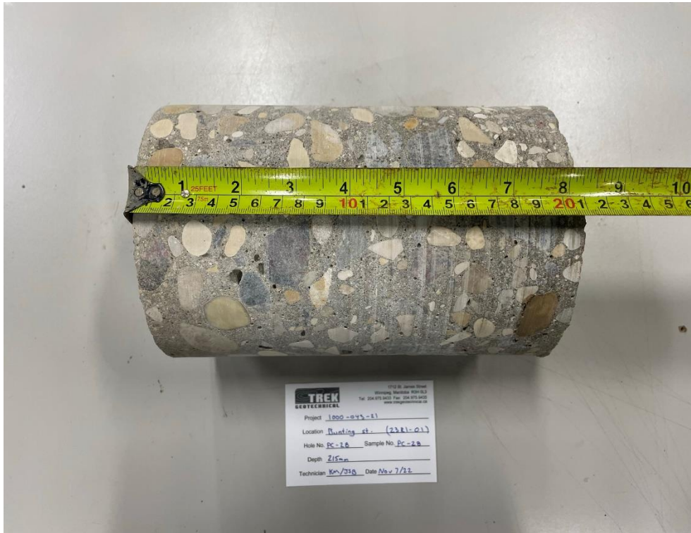
Photo 3: Pavement Core Sample PC-28
