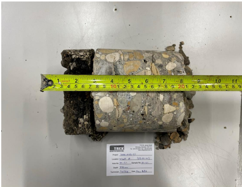
Photo 2: Pavement Core Sample PC-21
