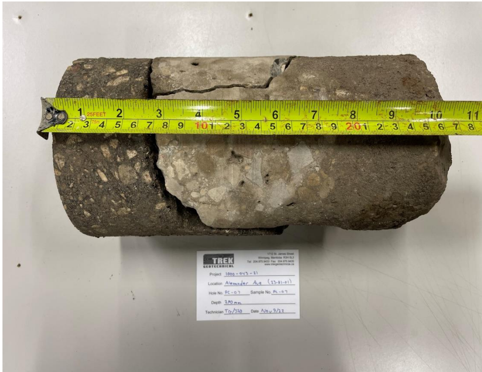
Photo 1: Pavement Core Sample PC-07
