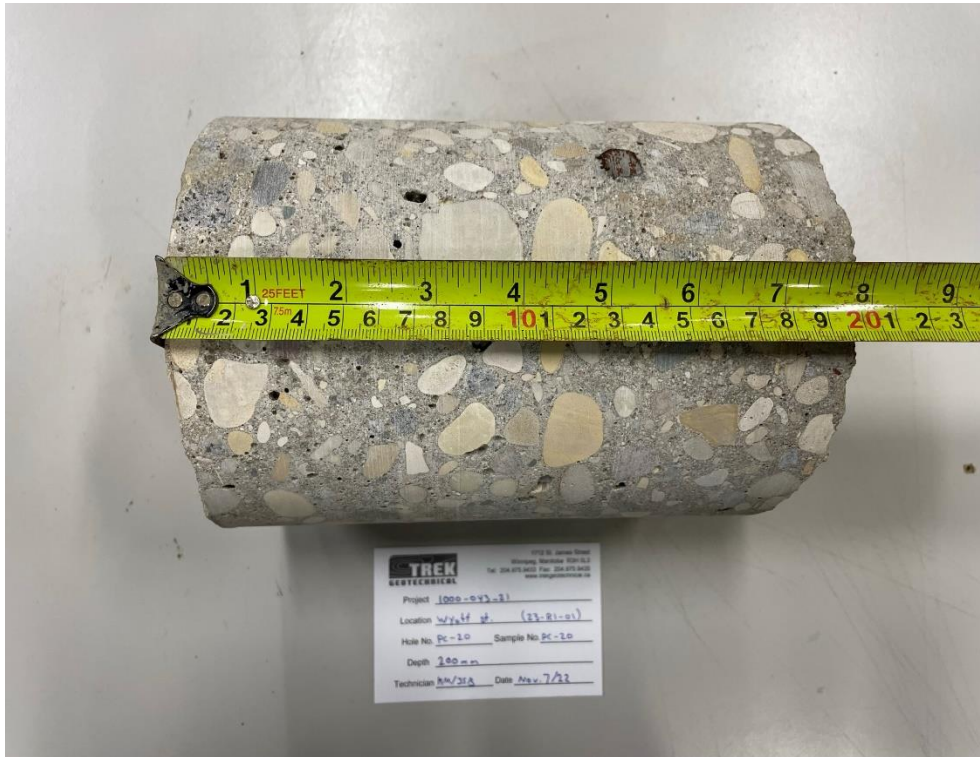
Photo 1: Pavement Core Sample PC-20
