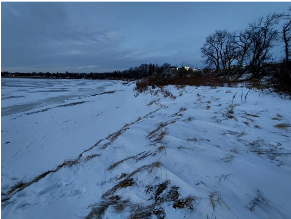
Photo 24: Looking downstream at toe of riverbank (water approx. 222 m) (December 1, 2022)
