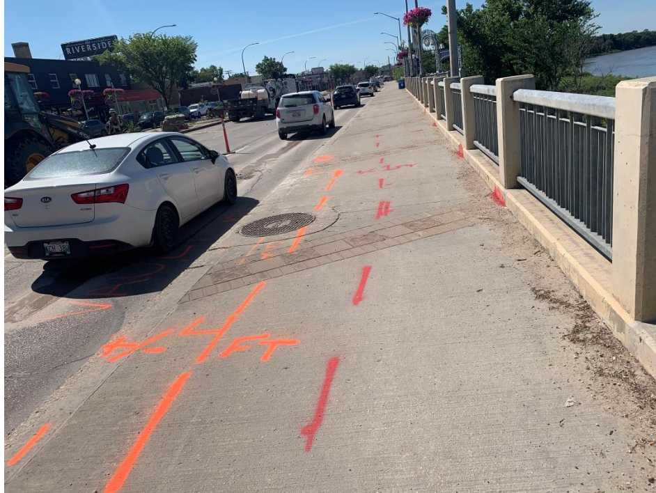
Photo 5: Looking south on St. Mary's. Utilities marked out on sidewalk (July 29, 2022)
