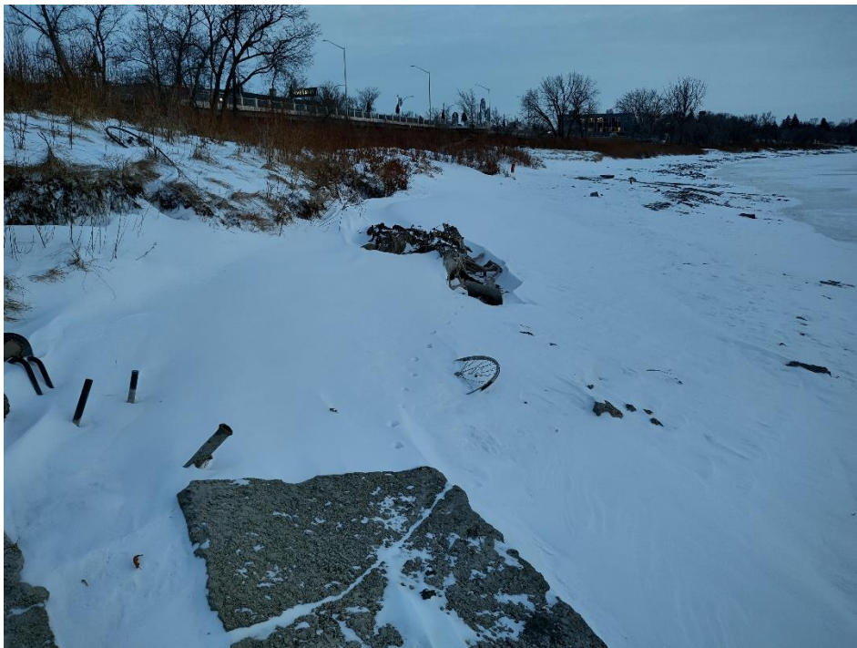
Photo 22: Looking upstream from old concrete block (to be removed). (December 1, 2022)
