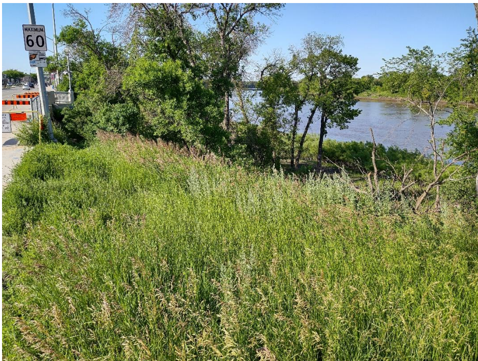
Photo 10: Potential site access. Looking upstream at the top of the bank showing the barricaded failed sidewalk (July 12, 2022)
