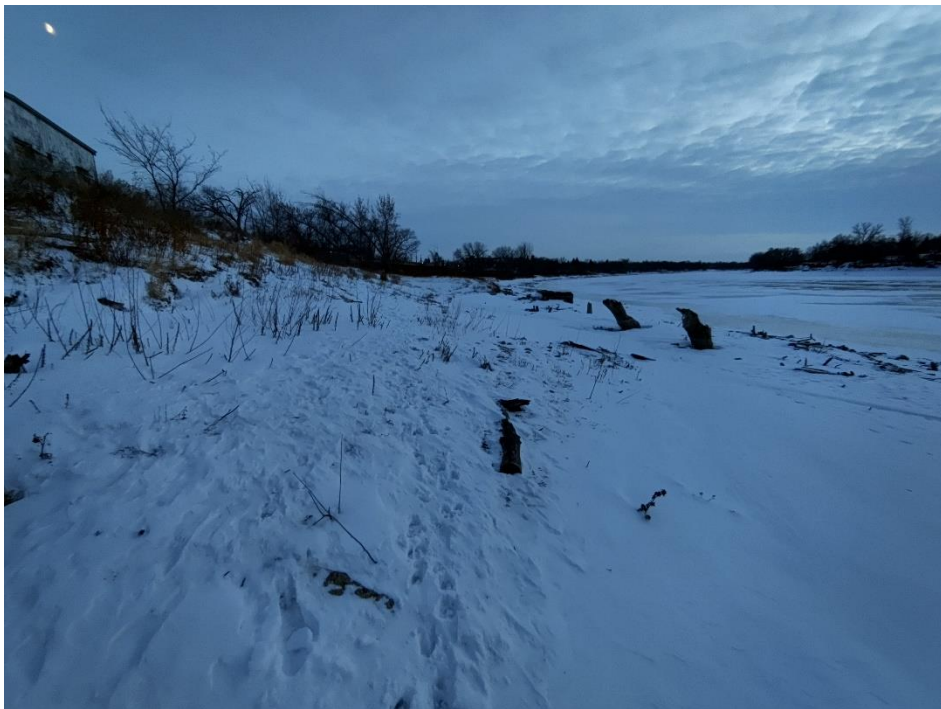
Photo 20: Looking upstream from bottom of construction access ramp. (December 1, 2022)
