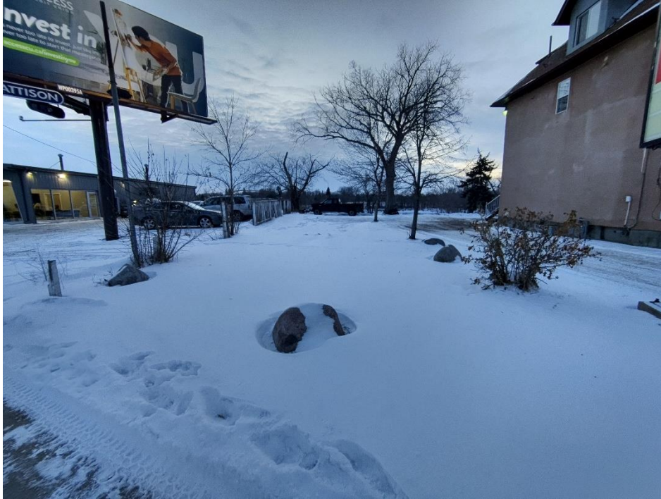
Photo 17: Location of top of construction access ramp at 480 St. Mary's Road. (December 1, 2022)
