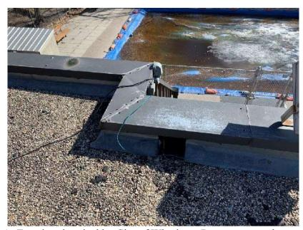
Fig. 8: Roof-A: Exterior electrical by City of Winnipeg. Parapet tops to be re-sloped back to roof a min. of 2%.
