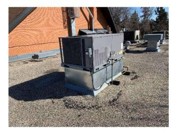
Fig. 5: Roof-A: Remove capped curbs & infill decking as required. Raise & reset mechanical as required.
