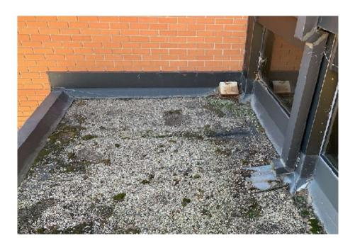
Fig. 11: Roof-B: Save splash pans for re-use. Modify & seal new reglet flashing(s) as required.
