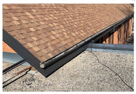
Fig. 3: Roof-A low-slope inset at steep-slope overhang to be boxed-out, insulated fully with batt insulation & sheathed to facilitate SBS roof assembly up-stand stripping.
