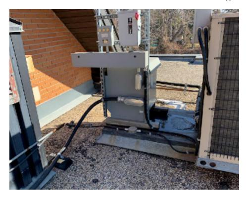
Fig. 7: Roof-A: Modify & raise platform curb including electrical & mechanical to facilitate min. 8 above new roof height.
