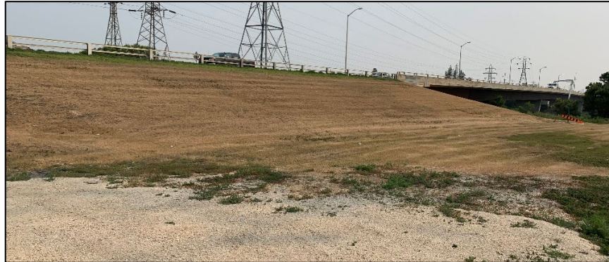
Photograph 1: Facing northeast from D'Arcy Pumping Station
