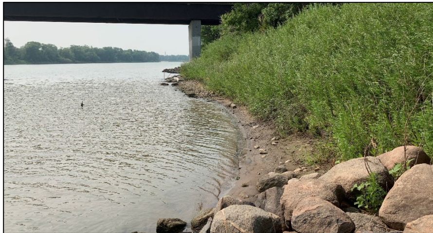
Photograph 2: Facing south (upstream) along the Red River near proposed outfall location
