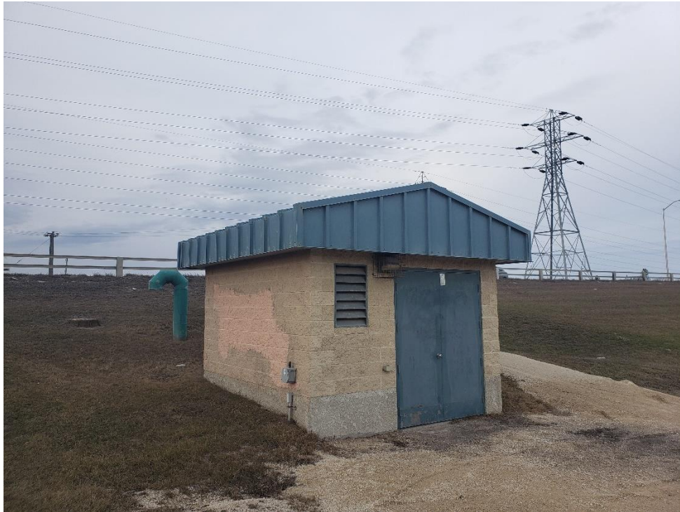
Figure 2-1: D'Arcy Wastewater Pumping Station
