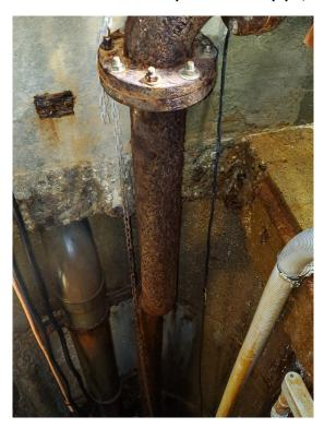
Figure 4 – Booster Pump Station sump pit, 100 mm discharge piping and bends.
