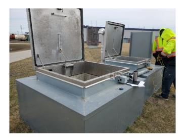
Figure 5 – Clearwell Sump Chamber
