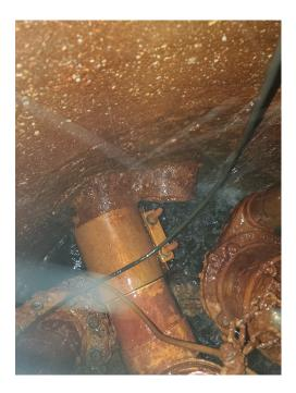
Figure 3 – Lower level of Booster Pump Station sump pit, 150 mm drains.
