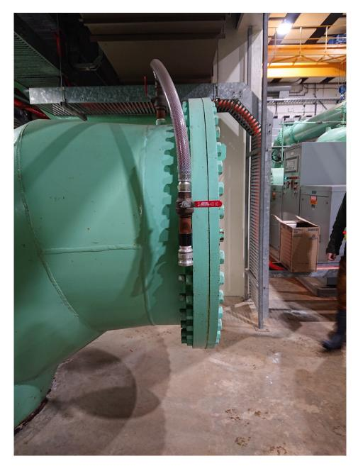
Figure 2: View of Pipe Bend Reducer and Blind Flange to be Removed
