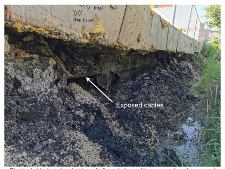
Photo 4: Undermined sidewalk foundation with exposed underground cables (looking southeast)
