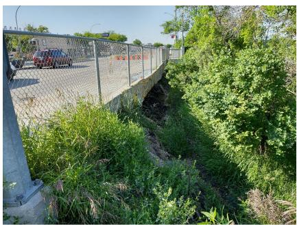
Photo 3: Section of undermined sidewalk foundation (looking southeast)
