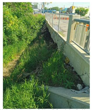
Photo 6: Undermined section of sidewalk foundation (looking north from north limit of the Old St. Vital Riverwalk)
