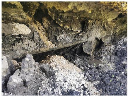
Photo 5: Exposed underground cables
