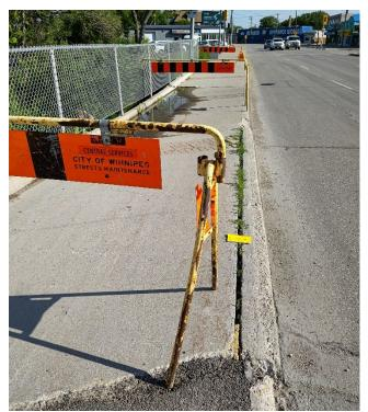
Photo 16: Curb separated from sidewalk slab (looking north)
