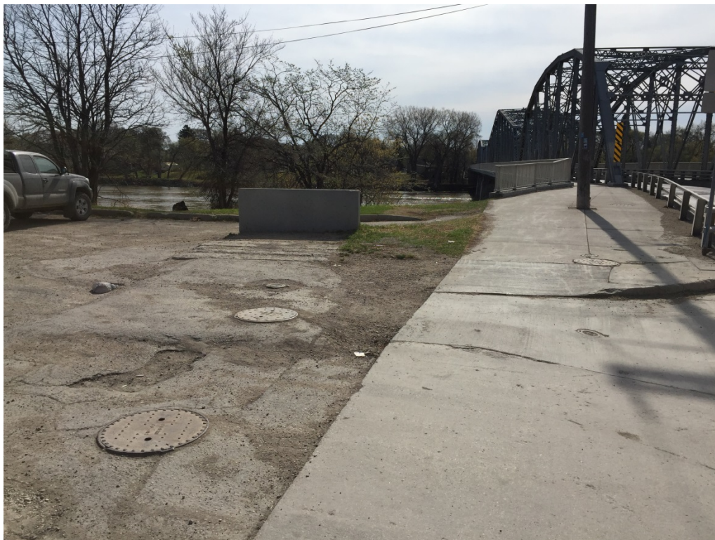
West Side – Existing tunnel shaft and valve chambers
