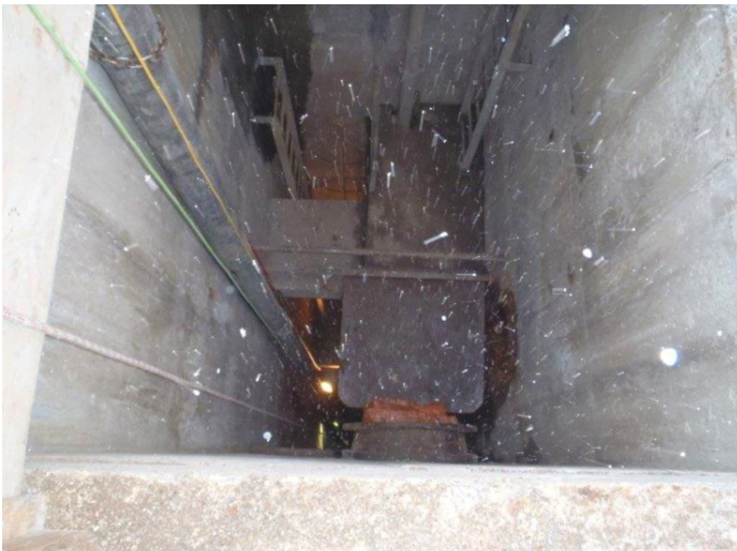
West Side - Existing tunnel shaft
