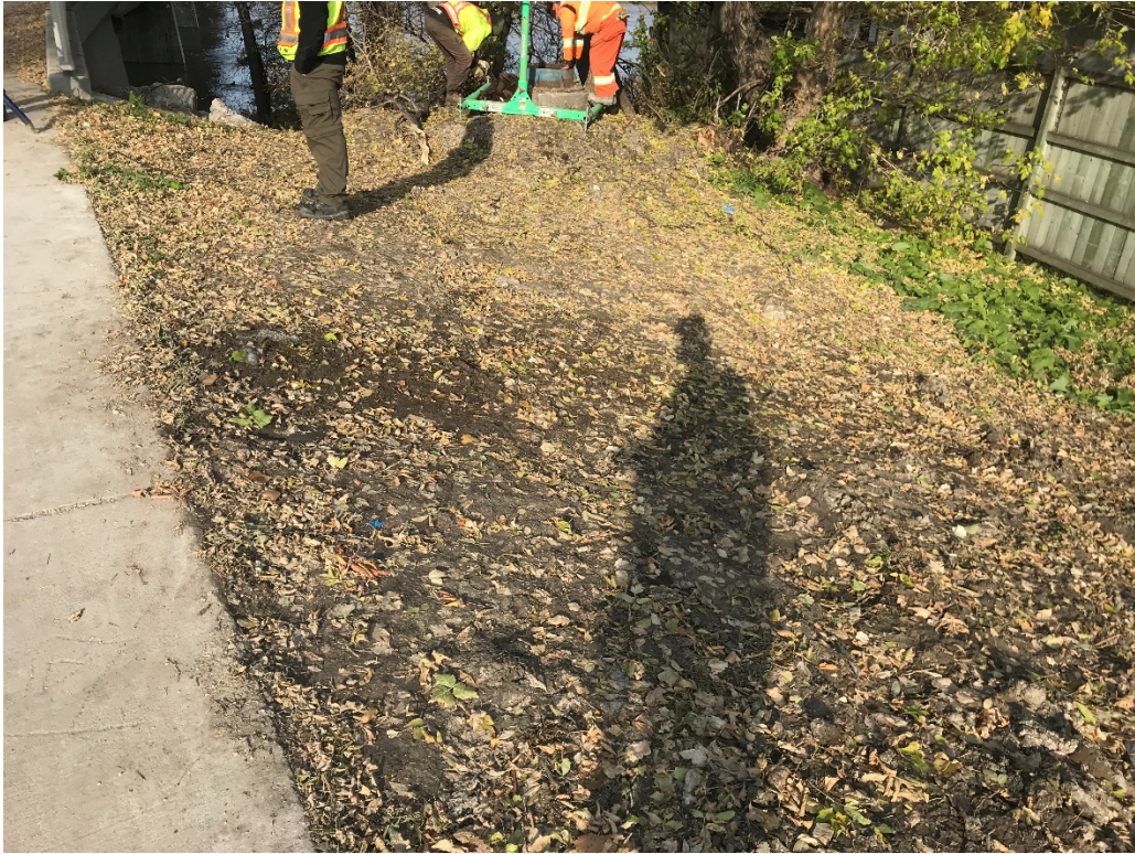
East Side – Existing valve chamber
