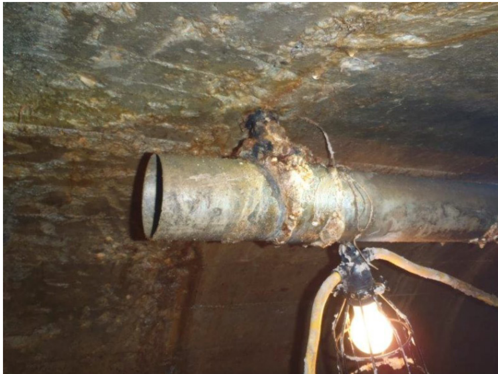
West Side – Existing tunnel ventilation piping (typ)
