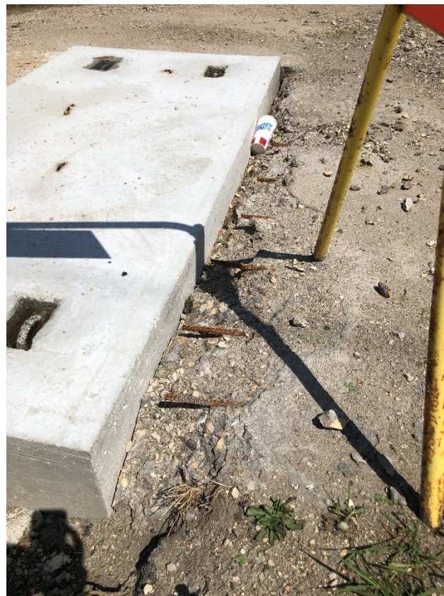
West Side – Existing Tunnel Shaft Roof Slab
