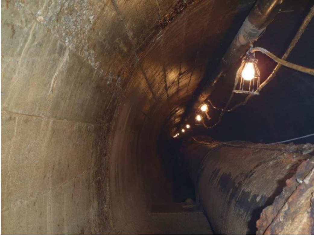
West Side – Tunnel and 600 mm feeder main
