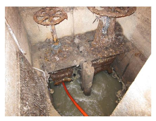
Figure 11 -Upstream siphon inlets, 300 mm siphon on left (to be lined), 450 mm siphon on right.
