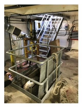
Figure 3 – Downstream siphon chamber at intermediate floor level. Stair access and access hole in intermediate floor.
