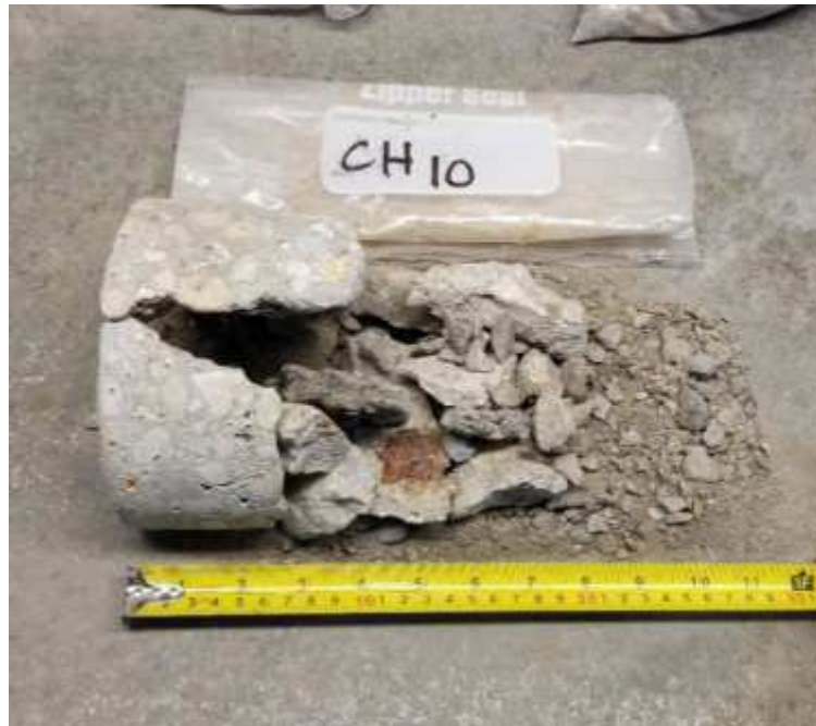
South bound transverse joint, Sta. 0+700
