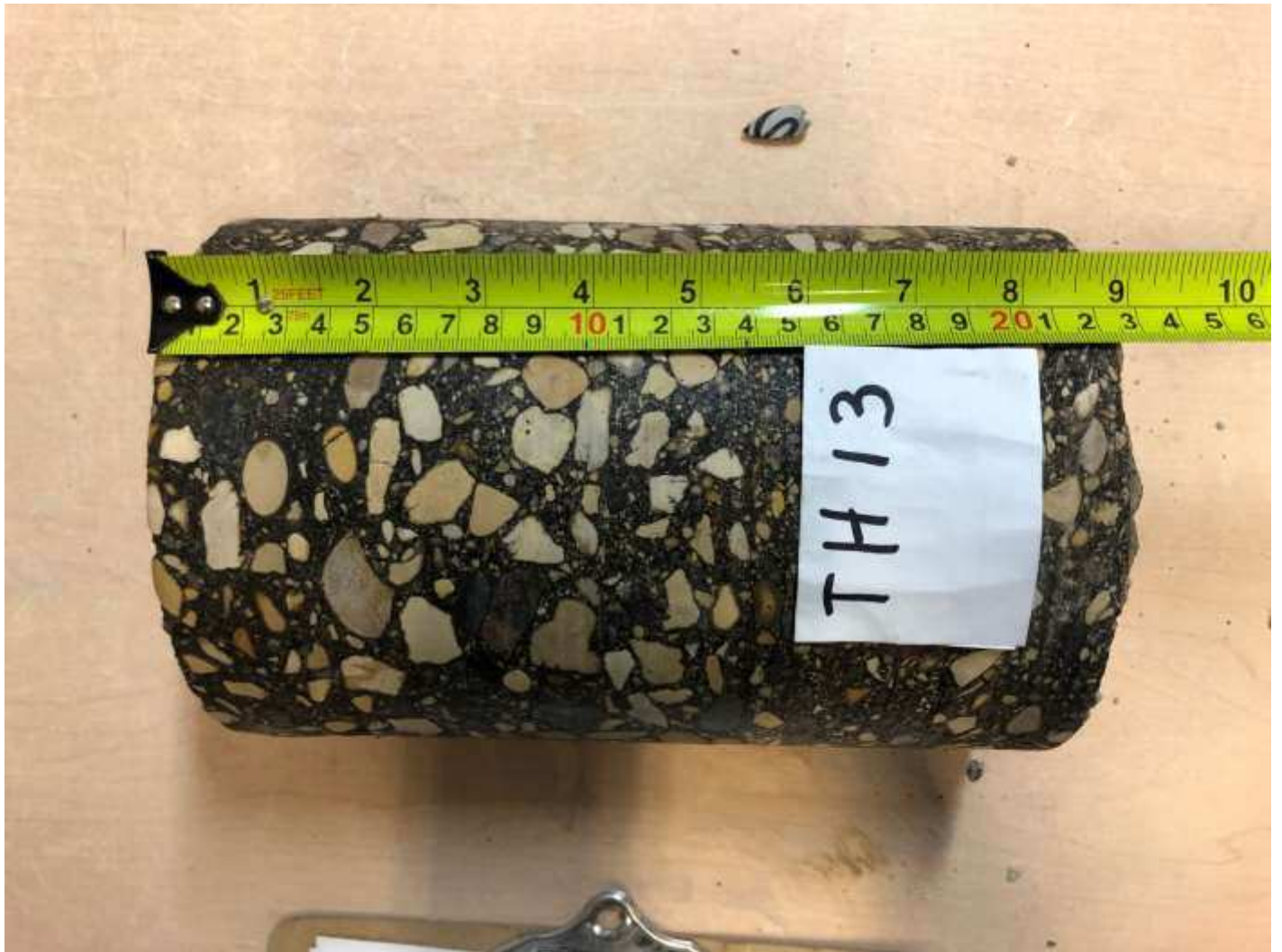
TH 13, north bound Sta. 1+250, concrete could not be recovered
