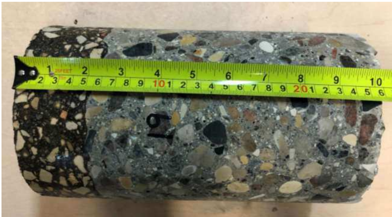
TH 9, north bound Sta. 0+547
