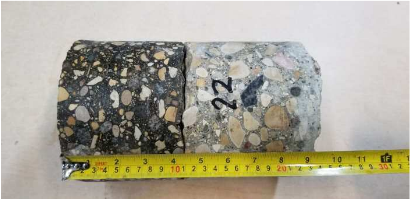
TH 12, north bound Sta. 1+000, lower part of concrete core could not be recovered
