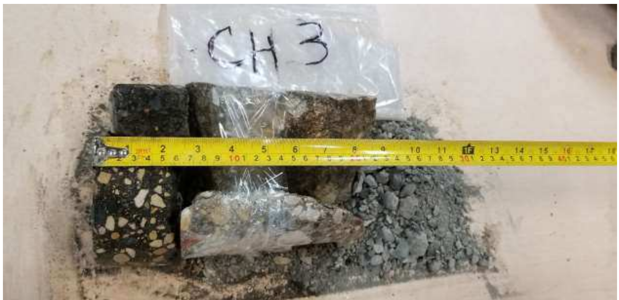
South bound transverse joint, Sta. 1+515
