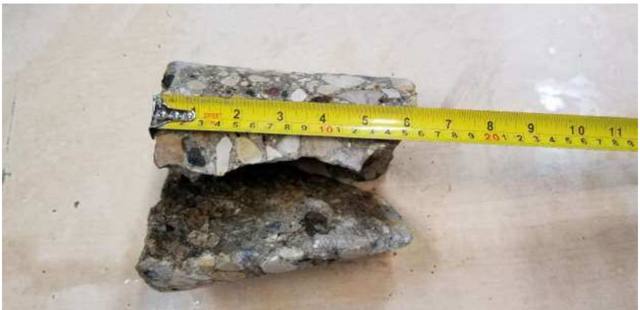
South bound transverse joint, Sta. 1+200
