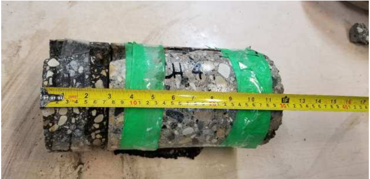
South bound transverse joint, Sta. 1+300
