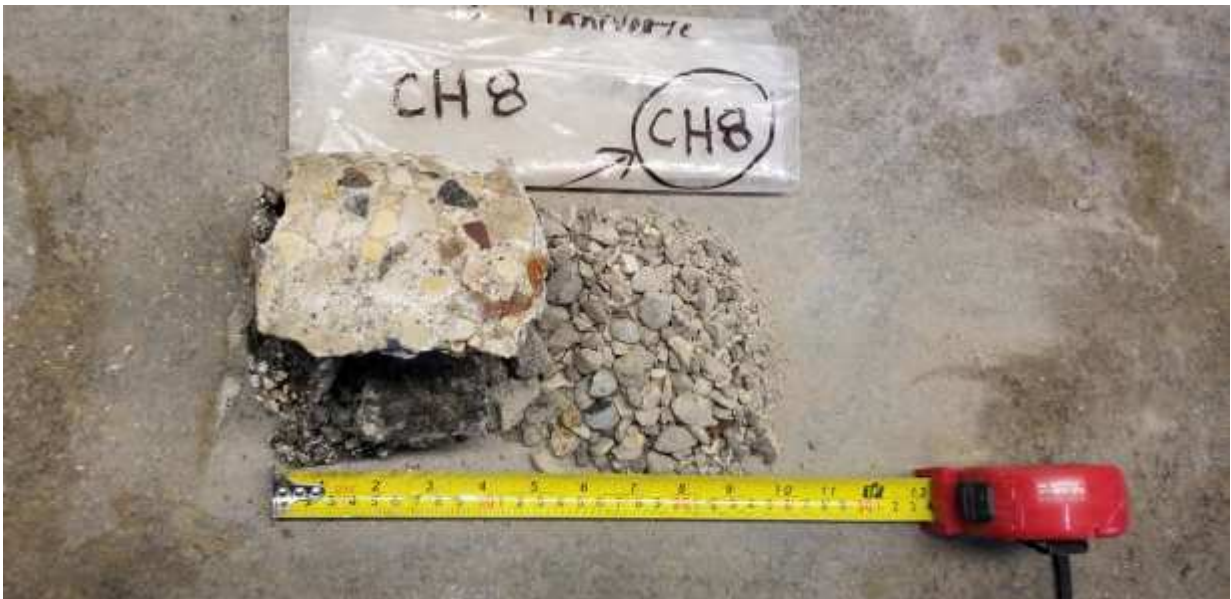
South bound transverse joint, Sta. 0+896
