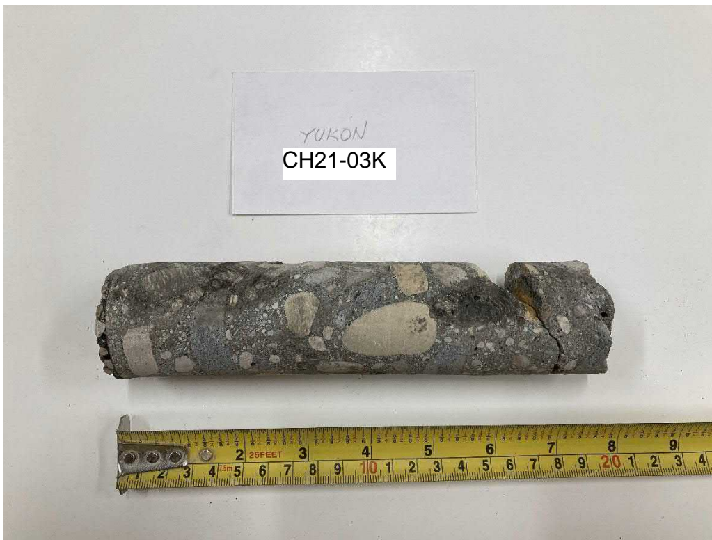
Photograph 18: CH21-03K - Yukon Avenue (Milt Stegall Drive to Empress Street)
