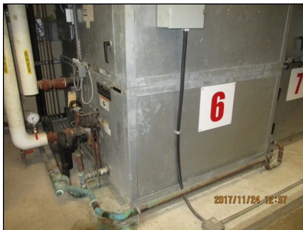
PHOTO 9 AIR HANDLING UNIT AH-6 AND REMOTE CONDENSING UNIT
