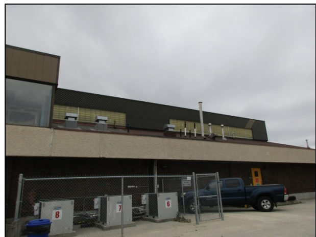
PHOTO 9 AIR HANDLING UNIT AH-6 AND REMOTE CONDENSING UNIT
